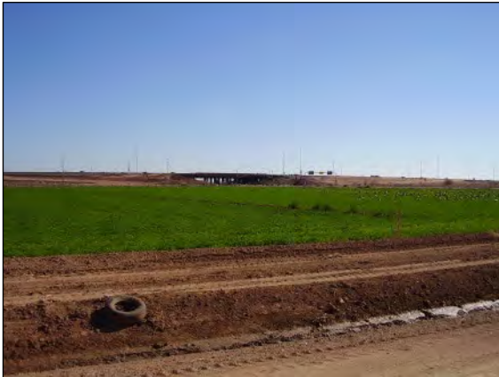
Typical ADOT overpass (0.25 mile away)
