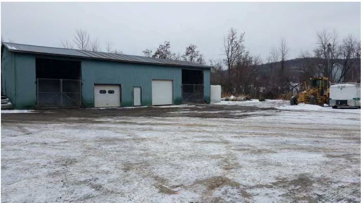
Photo 6: The south side of the large cold storage shed.
