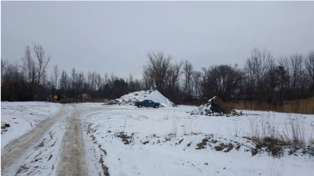
Photo 10: The northern portion of the Site facing north. The large soil stockpile just beyond the pickup truck was excavated from the St. Albans Core Lot Project. The excavator to the left of the soil stockpile is located on the “footprint” of the former Core Lot Project stockpile which was recently transported to a landfill. The smaller stockpile in the foreground was generated during water main breaks and other DPW projects and will be transported to the DPW fill site once weather permits.
