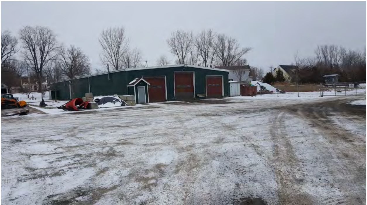
Photo 8: The east end of the main DPW building looking northwest. The small white trailer at the northeast corner of the main DPW building is used to store fuel for the small engines used by the DPW.
