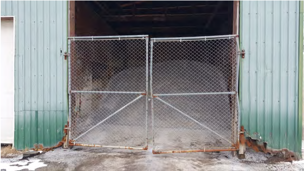
Photo 26: Salt storage in the large cold storage shed
