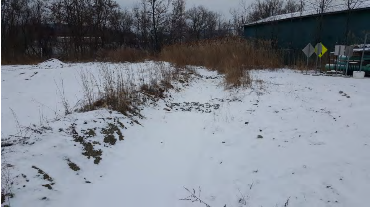
Photo 11: Drainage swale with check dams
