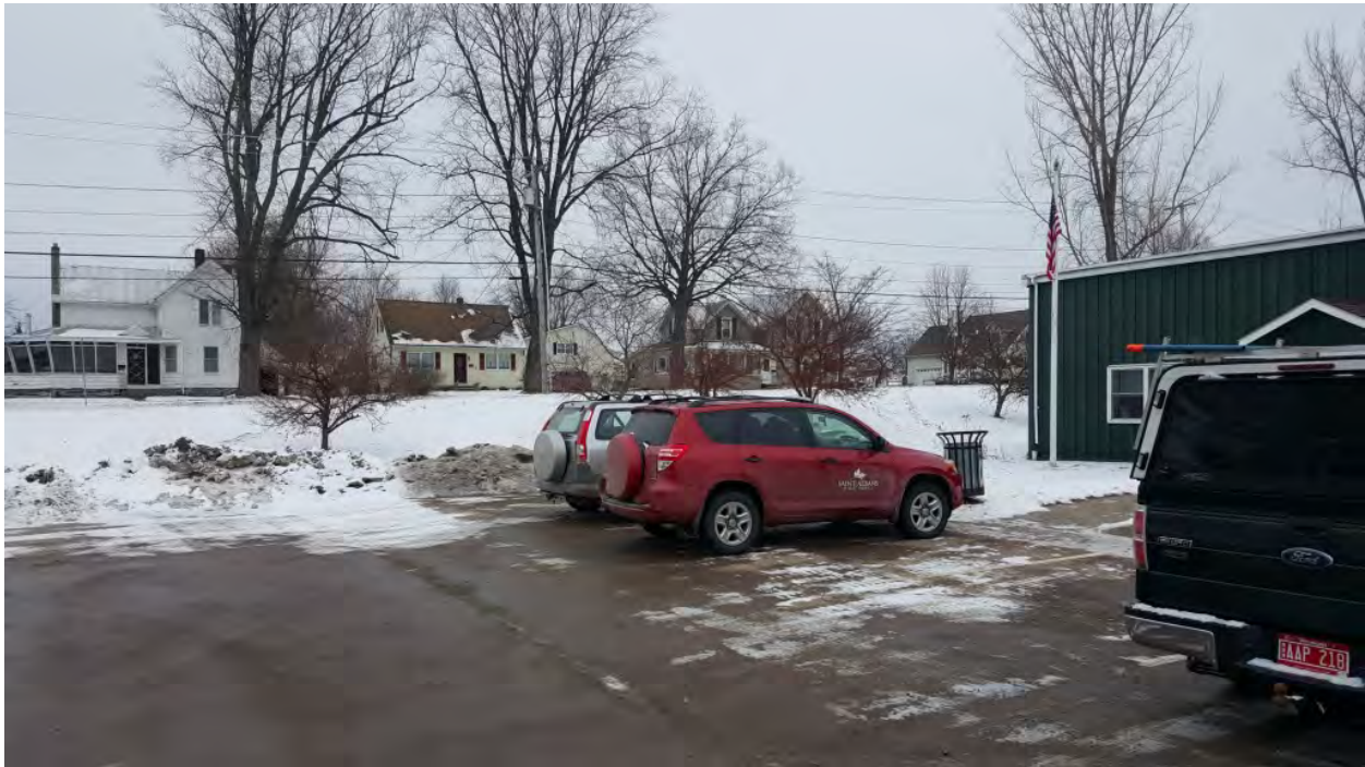
Photo 2: View of the south side of the main DPW building looking west. The telephone pole with the transformer visible in the background provides power to the main DPW building. This pole is not located at the Site according to information provided by Mr. Allen Robtoy.
