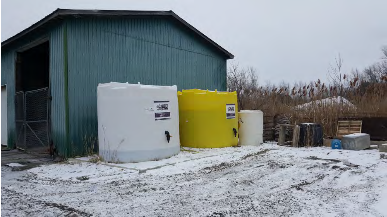
Photo 9: The tanks of deicing solution at the east end of the large cold storage shed.
