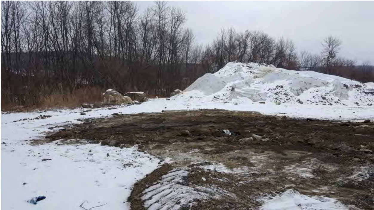
Photo 12: View of the Core Lot Project soil stockpile facing east. The other stockpile which was transported to the landfill was formerly located where the bare ground is visible.
