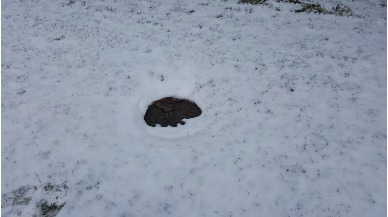
Photo 3: Sewer utility hole to the grit separator for the floor drains.
