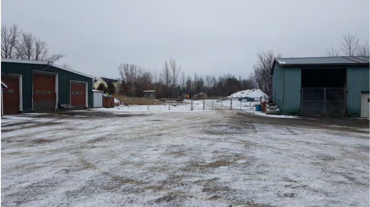
Photo 5: The view looking north between the main DPW building (left) and the large cold storage shed (right). The second storm drain is present to the left of the main DPW building. The gate to the northern portion of the Site is visible at the center of the photograph.
