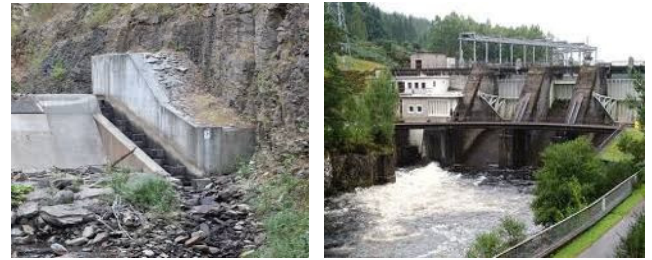
Fig 10. The SHP Racaciuni before, and after rehabilitation
