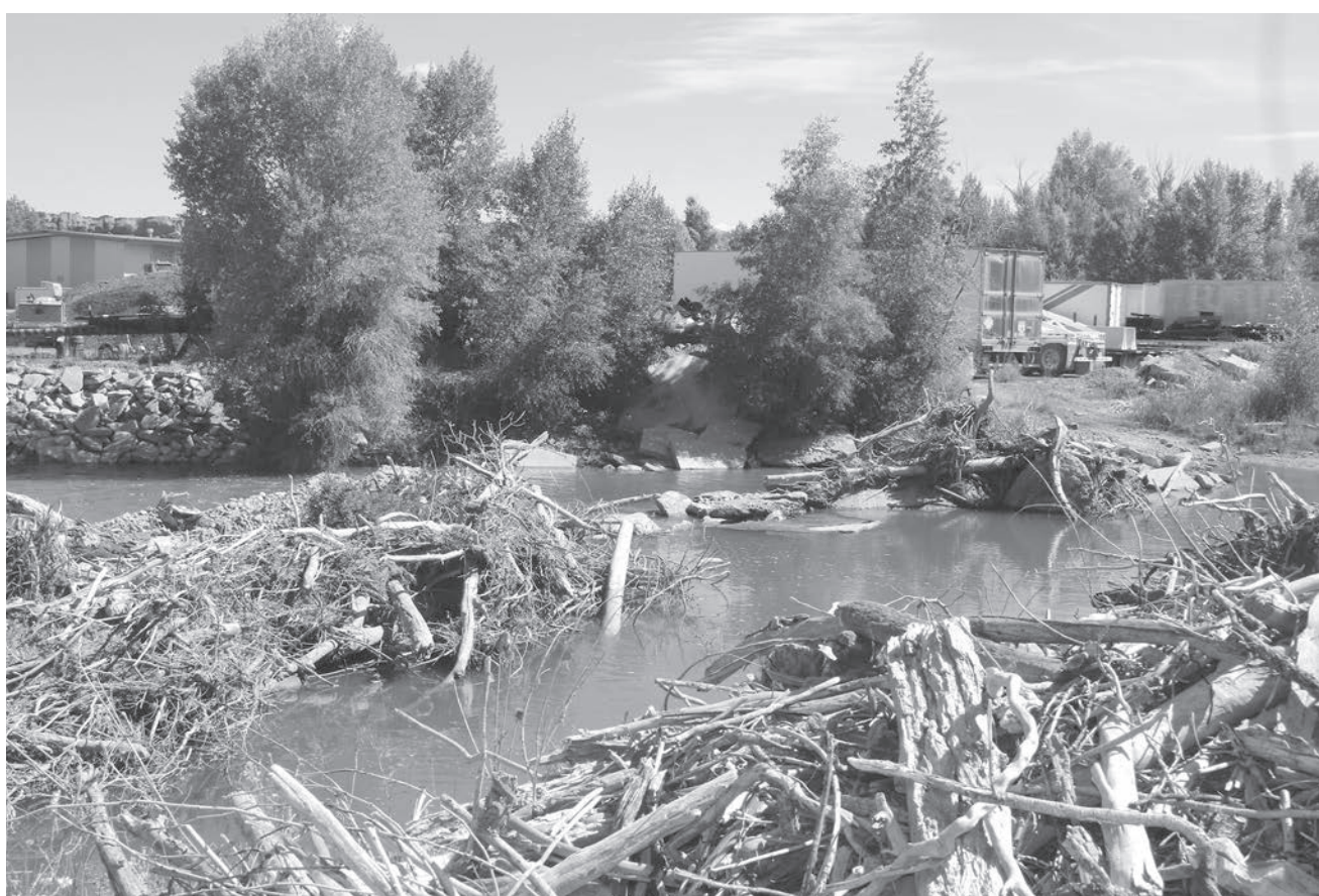
Pictured is the current dam created by landowners to direct water into canals at the Sims Creek slough along the Bear River. A diversion dam will be built in 2024 using the same methods that were used at the Evanston dam project. (UINTA COUNTY HERALD/Kayne Pyatt)
