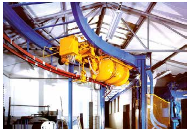
Feed and control of a concrete skipper
