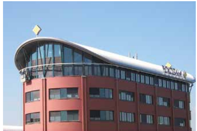
Curved installation for window cleaning equipment
