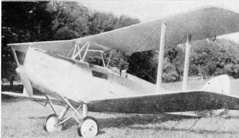
Above: Nigel Norman's G-AAHI flew in the 1930 King's Cup as a single-seater with a hood over the pilot's cockpit faired right back to the tail and with the front cockpit covered over. It also had stub exhausts fitted. (via Jack Meaden)
