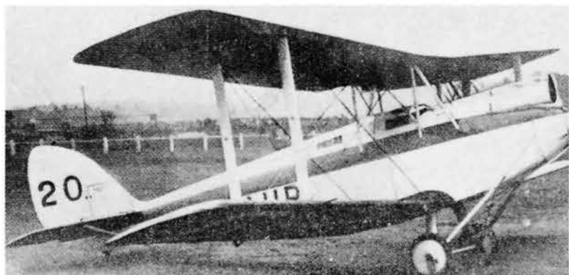
Above: H.S.Broad's low-top enclosed Moth G-AAHR in its initial racing configuration with straight-axle undercarriage and small wheels. Flown from the front cockpit it was later converted to a large wheel divided undercarriage. (Aeroplane via Jack Meaden)
