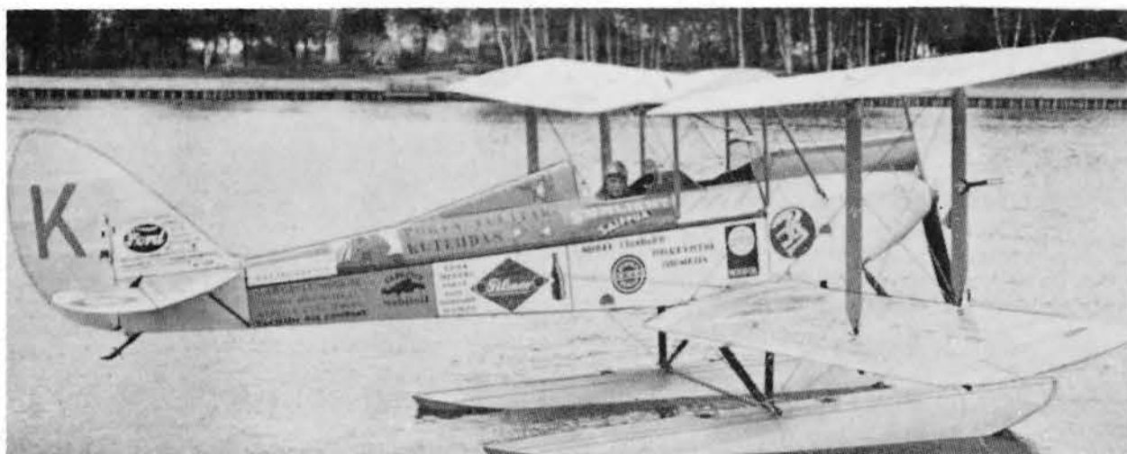
Above: H.S.Broad's low-top enclosed Moth G-AAHR in its initial racing configuration with straight-axle undercarriage and small wheels. Flown from the front cockpit it was later converted to a large wheel divided undercarriage. (Aeroplane via Jack Meaden)
