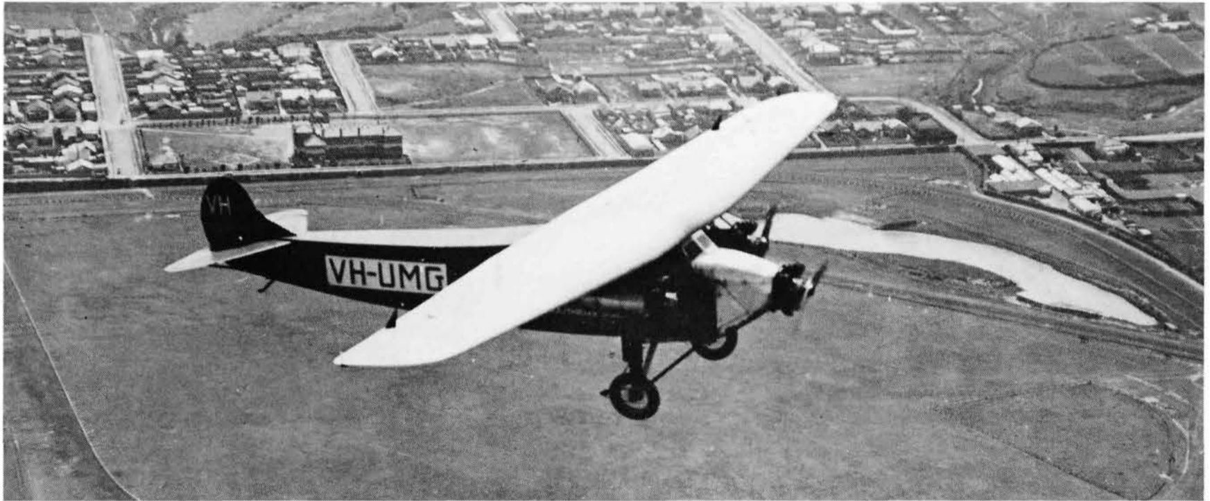
Above: VH-UMG "Southern Star" c/n 230 was the second of 5 Avro Tens for Australian National Airways. In this view from above, the 2 feet thick straight centre section of the Fokker wing is seen with the pilots' cockpit under the leading edge. The projection behind the near wheel is a scraper to prevent mud being thrown up by the wheels on the grass airfields of the time. These replaced the mudguards fitted above the wheels on this aircraft and on VH-UMI and VH-UNA in Australia. (via Jack Meaden)
