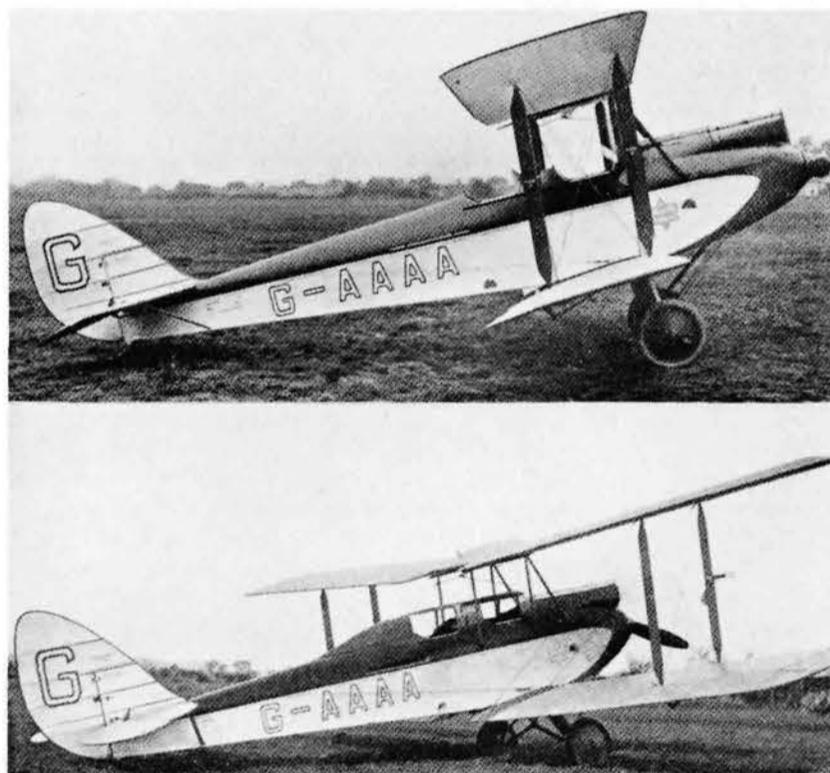
Above: Upper: G-AAAA seen in new condition as a standard DH.60G open cockpit Gipsy Moth, a configuration to which it returned after trials and demonstrations as the coupe Moth prototype. Lower: G-AAAA with prototype coupe hood fitted. The quadrant ASI can be seen projecting from the front right-hand interplane strut. (via Jack Meaden)
