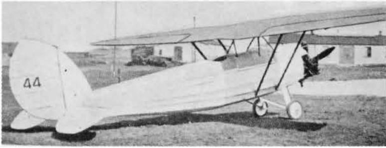
Top: The Clarke Cheetah G-AAJK c/n CC.1 (35hp Blackburne Thrush 3-cylinder radial) used a number of DH.53 parts and was designed as a convertible biplane/monoplane, the lower wing (from the Halton Mayfly G-E800) being removable. (JM)
