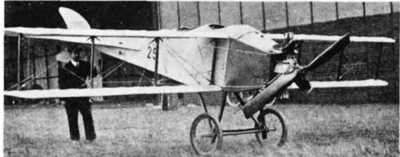
The third design, called the Piggott Military Biplane, (above) was the one we illustrated on p90/58. It was entered for the 1912 Military Trials at Larkhill as "29" but while being taxied by Parr it was damaged after hitting an obstruction and took no part in the Trials. It was underpowered with its 35hp Anzani 3-cyl radial engine and there is no record of it being flown successfully. It is believed that the Piggott machines were all disposed of in 1912.
