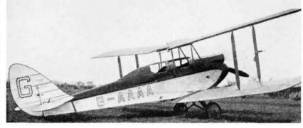
Above: Upper: G-AAAA seen in new condition as a standard DH.60G open cockpit Gipsy Moth, a configuration to which it returned after trials and demonstrations as the coupe Moth prototype. Lower: G-AAAA with prototype coupe hood fitted. The quadrant ASI can be seen projecting from the front right-hand interplane strut. (via Jack Meaden)
