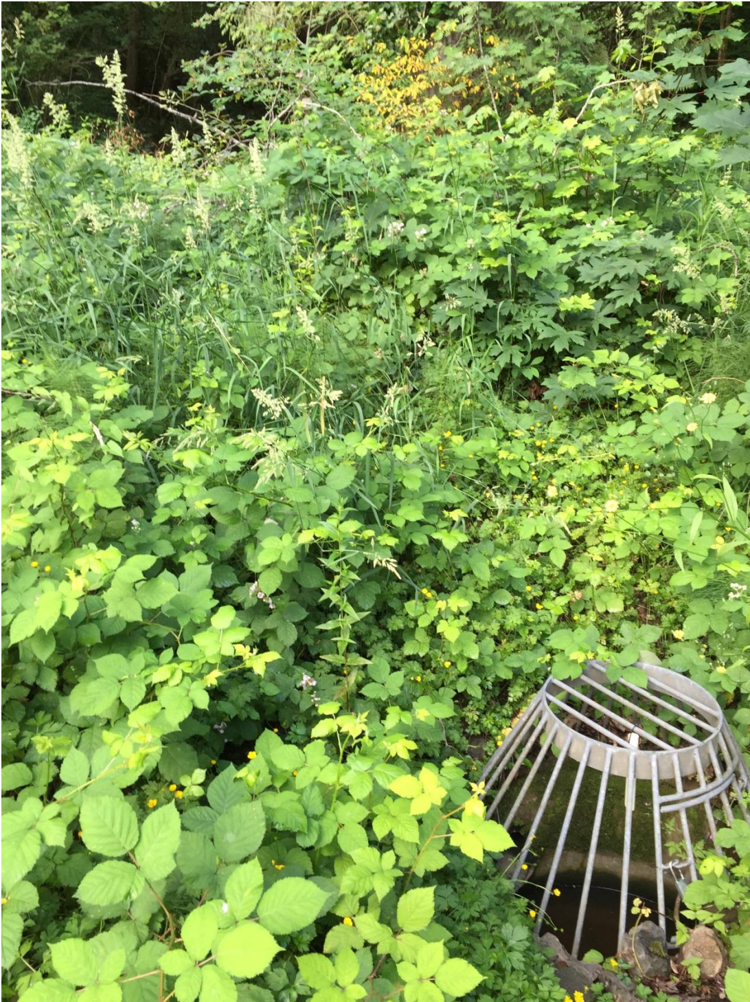
The existing type 2 catch basin with birdcage which is the collection point of NDA 2.
