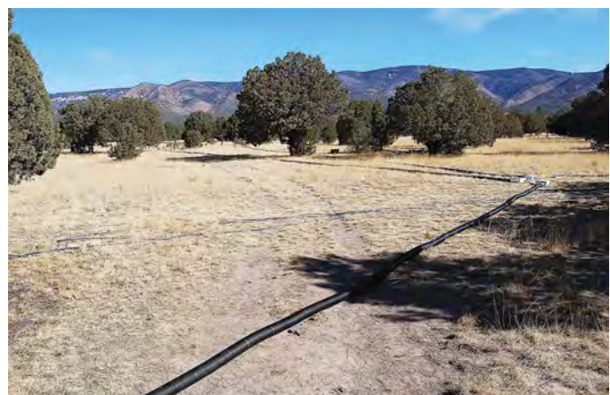
Fig. 6. Site view of station BACA, showing 60-m long optical fiber array elements.
