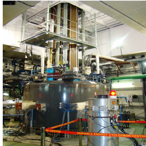
Figure 1: The K500 superconducting cyclotron
