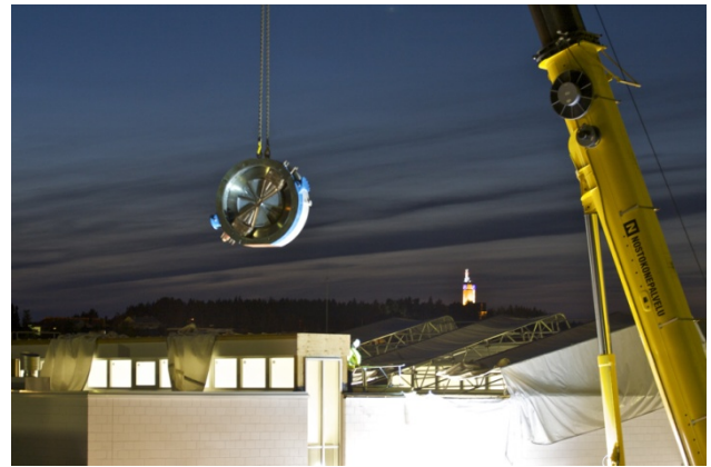
Figure 1: The first half of the MCC30/15 cyclotron is being lifted into the cyclotron cave.
