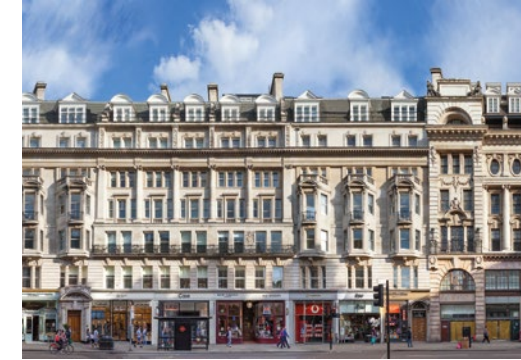
PICCADILLY BUILDINGS, SW1 Let to Cath Kidston, Richoux, New & Lingwood, Alfred Dunhill and Wiltons Restaurant Size: 187,100 sq ft, mixed-use
