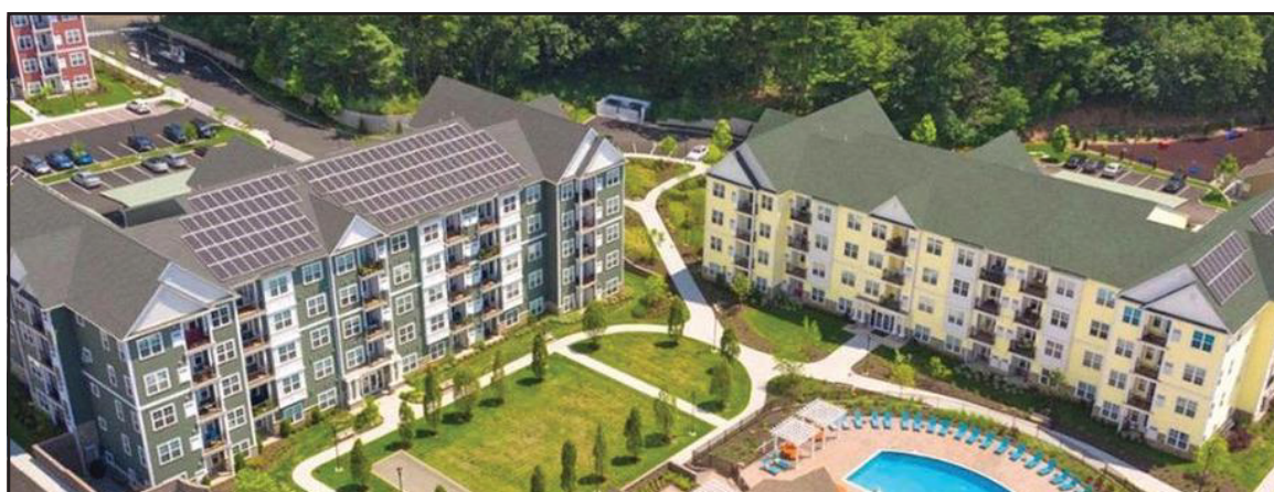
Canal Crossing at Whitneyville West - Hamden, CT
