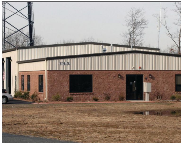
153 James P. Murphy Highway - West Warwick, RI
