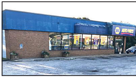
THE FORMER NAPA AUTO PARTS STORE IN WESTERLY, RI A 9100 SF VACANT STAND-ALONE BUILDING ON 1.5 ACRES SOLD FOR $93 PSF
