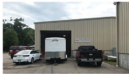
440 Dry Bridge Rd., North Kingston - Only triple unit in industrial condo complex, 3 units, 3600 sf, no walls or columns between, 12x14 OH door facing road for easy access. Many uses including indoor cultivation, 200 amp - 3 ph service, 18-20' ceiling ht - easily mezzanined for add'l sf. $450
