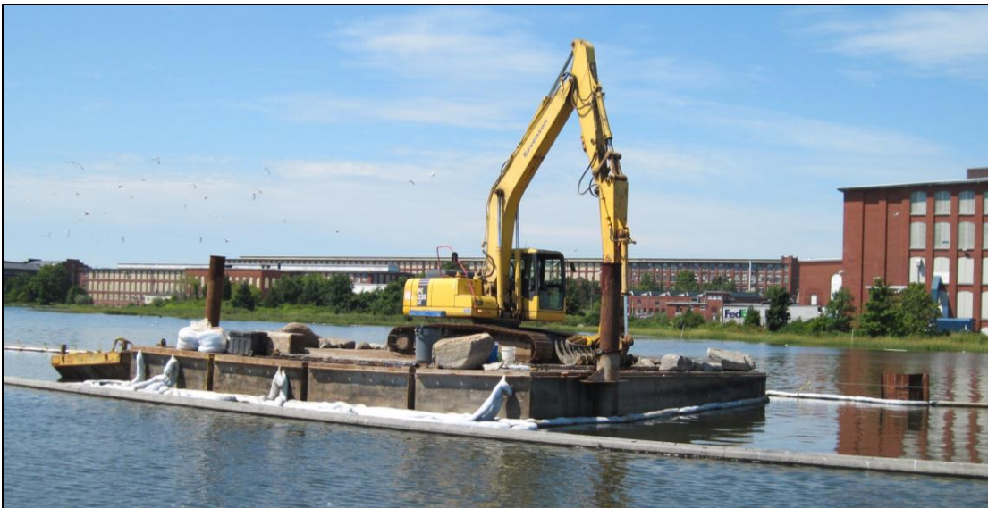
Figure 9. Debris Removal Excavator and Debris Storage Scow
