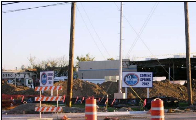
Kroger at corner of Maple and Medical District Drive – under construction
