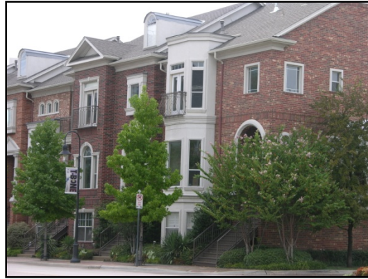
Camden Phase II - 17 Town Homes
