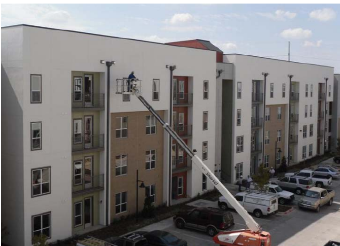
The Taylor Farms project under construction
