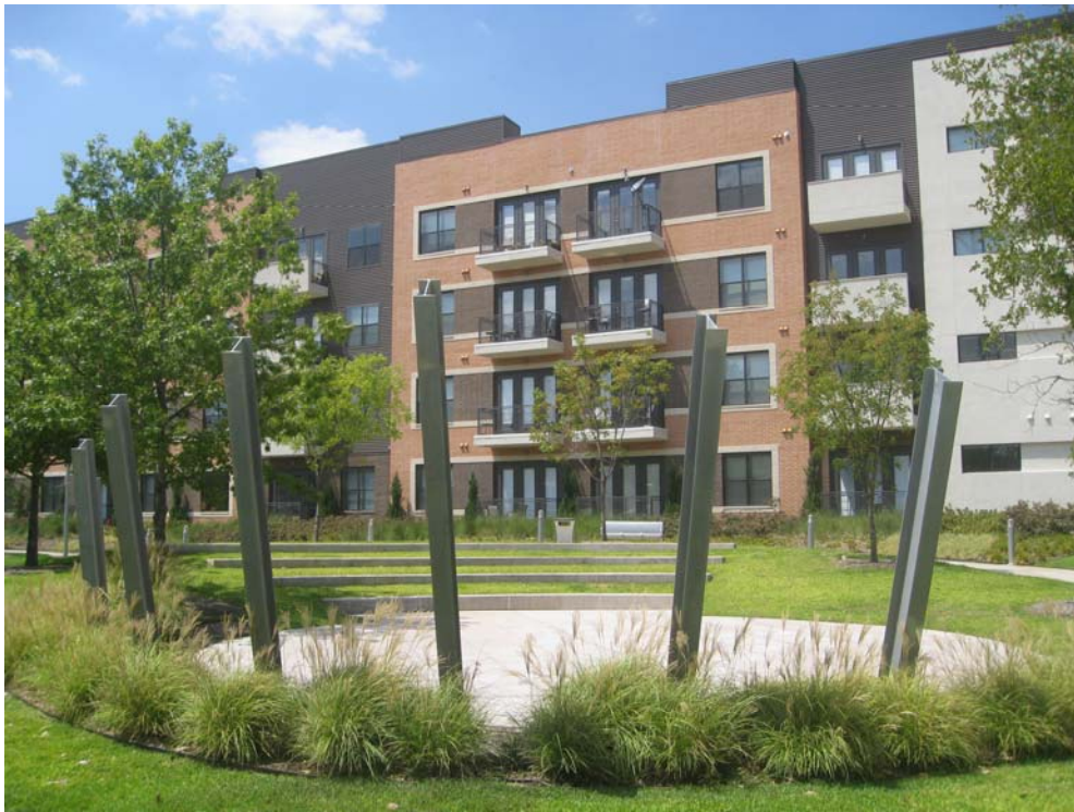
Alta 1900 Lofts and civic plaza along Oak Lawn Avenue at Hi Line Drive,
