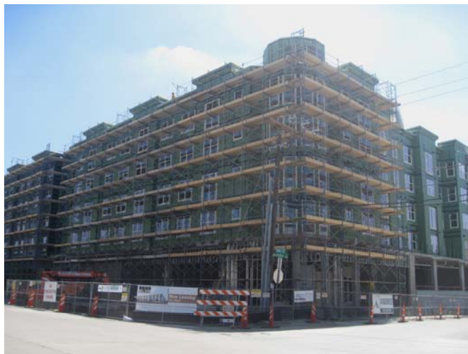
The BLVD (former Shamburger warehouse site) under construction
