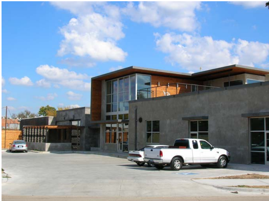
"The Olympia Arts" Building on Eastside Avenue
