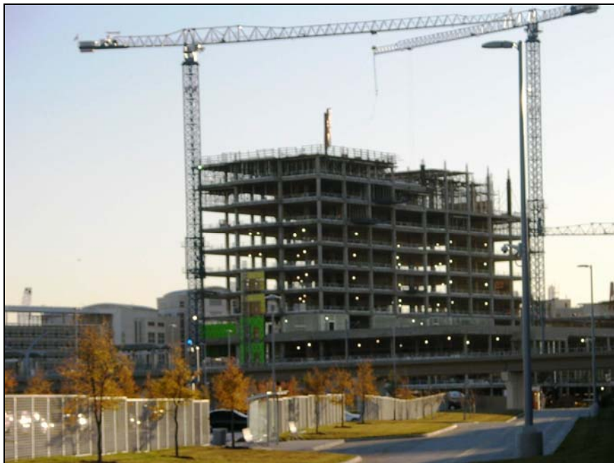
New Parkland Hospital - under construction
