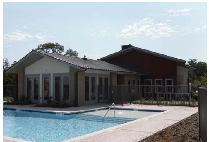
The Taylor Farms project's business center and swimming pool
