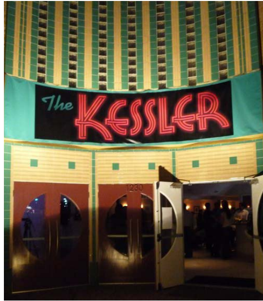
Kessler Theater Renovation Project: the renovated exterior façade, showroom and bar.
