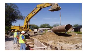
**Project Description:** The Southmont area business district sewer system improvements is to develop the infrastructure necessary for economic growth and development in the Southmont area. The project includes 6,400 LF of 8" gravity sewer, forcemain, manholes, air relief valve in
