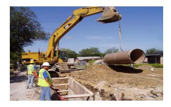
Project Description: Sanitary sewer extension and improvement on Highway 150 at Northwest Elementary School. This project includes 8" PVC Sewer and 8" DIP Sewer. It also includes manholes, service stub and clean out, stabilization stone and erosion control. Engineering fees and easement acquisition are included in the cost of this project. This project develops the infrastructure necessary for economic growth.
