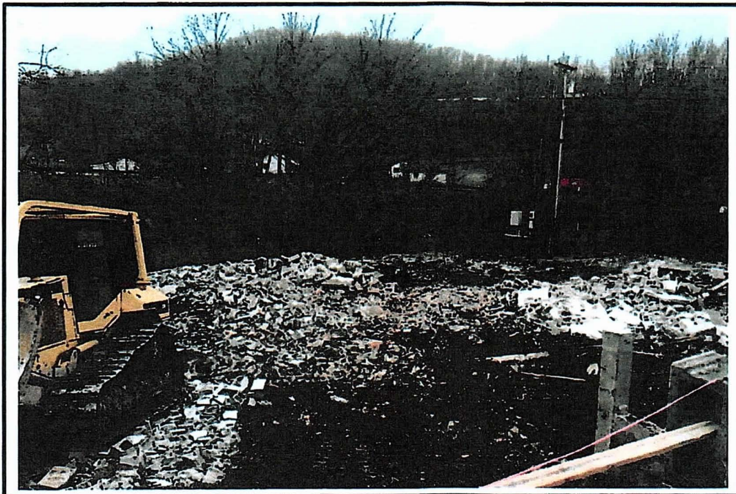
1/5/2017 – Mainline LLC bulldozer completing demolition.
