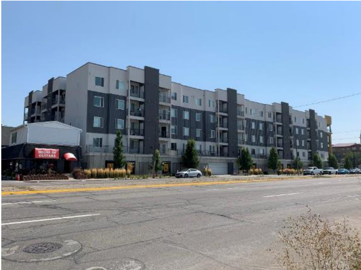
View of Moda Granary Place to the southeast
