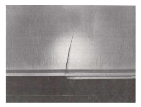
Figure 3-12 Fatigue Crack at Cover Plate Detail
