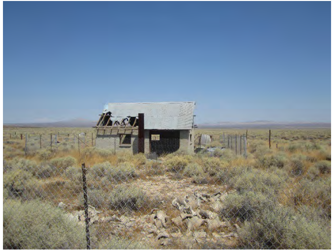
View of abandoned structure adjacent to the southwest corner of the Project Site.
