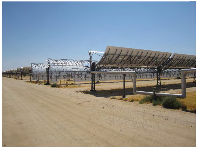
View of the SEGS IX solar fields adjacent to the south of the Project Site.
