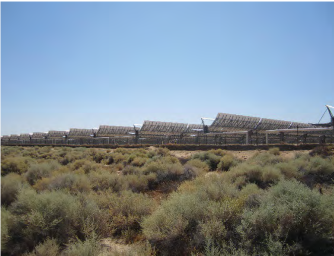
View of SEGS IX solar fields adjacent to the south of the Project Site.
