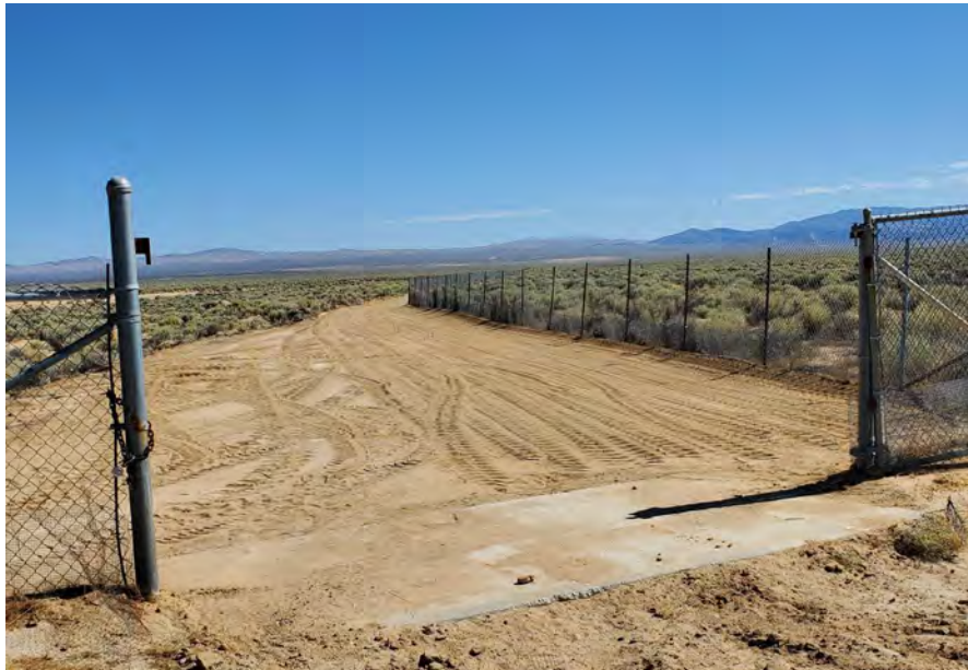
Gated entry point with exclusionary fencing
