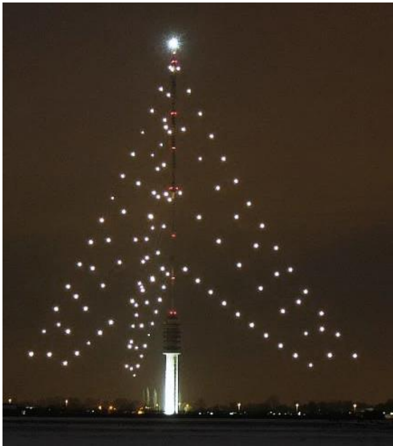
The Gerbrandy Tower in IJsselstein, The Netherlands, is used for directional radio services and for FM- and TV-broadcasting. The tower with guyed aerial mast is 375 meters high.
