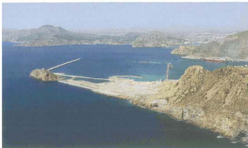
New works at Esperanza – from SE
