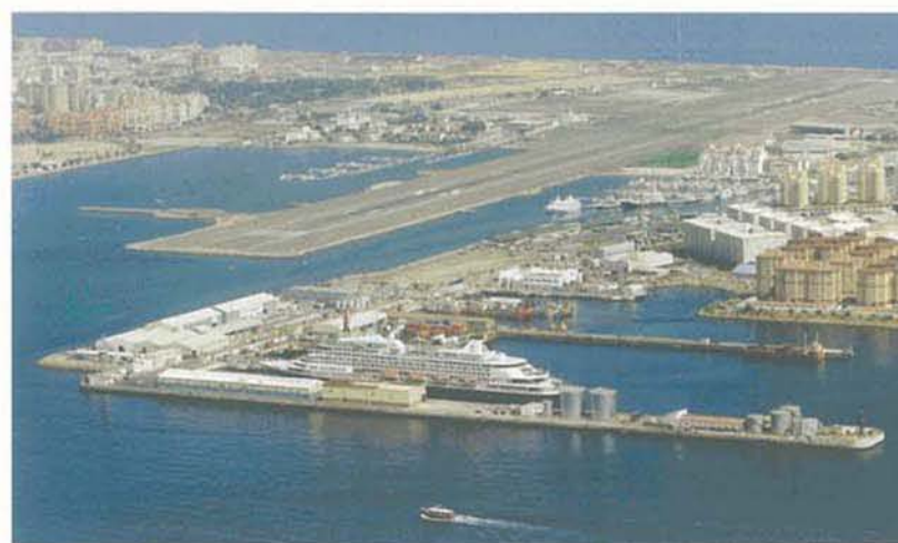
Gibraltar showing new construction for Sheppards marina north of the runway
