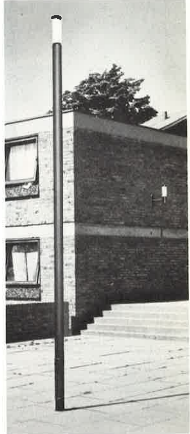
QG7 EFO1080.E27 lantern on QLC 1540/G7 column and QPRK/1100 wall bracket
