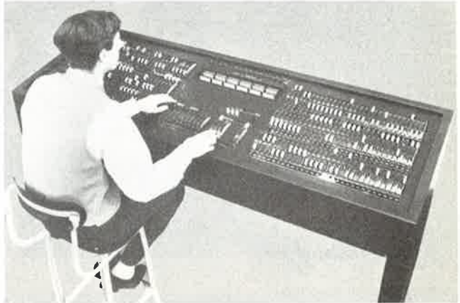
PM System at the Malakoff Theatre Paris.
