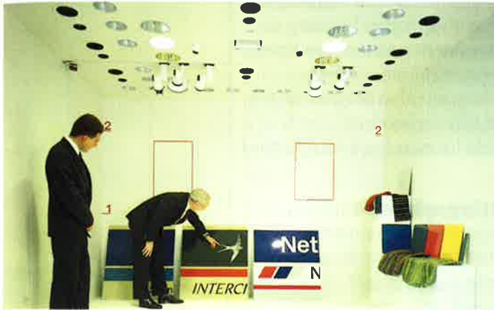
The Centre contains a Lita 'cube' – a small, bare room whose ceiling is covered with downlights. It demonstrates the precise effects produced by various luminaires and display lamps of different beam angles.
