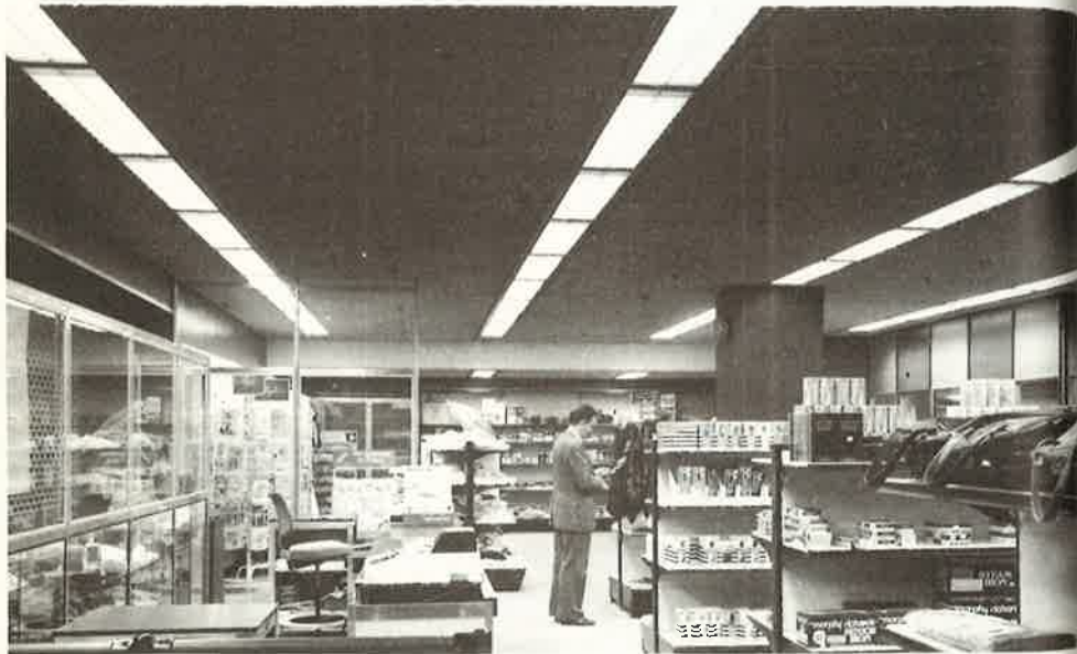
Air handling luminaires in Shell Centre Supermarket, London.
