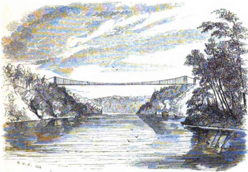
THE SUSPENSION BRIDGE, FROM THE MAID OF THE MIST
