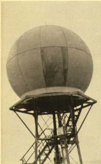
Above the dome is a lightning arrester and an obstruction light. The tower frame and lightning arrester are solidly grounded to the building.
