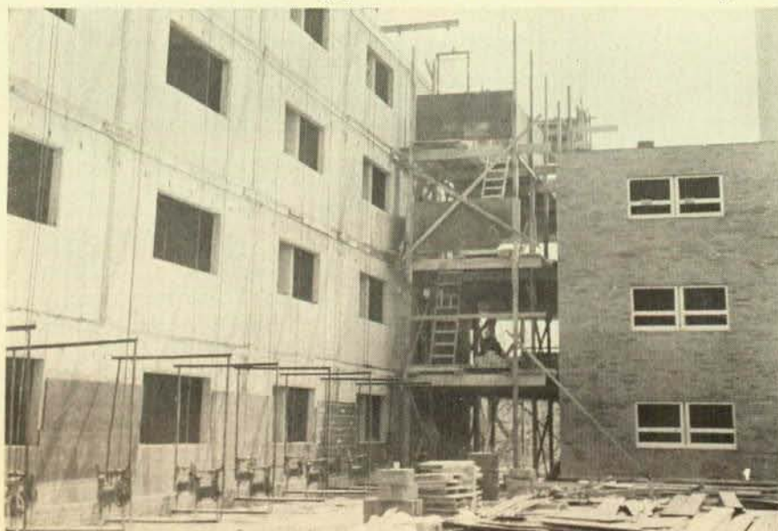
These members of Local 43, are wiring the new addition to the motherhouse of the Sisters of St. Francis in Syracuse, N.Y. This is one of the first multi-storied construction jobs of tilt-up precast walls. At right above are Foreman Carl Bauder and Brother Jerry Hart and below are Brothers Sam De Fonde, Willis Reese and Rovell Fuller.
