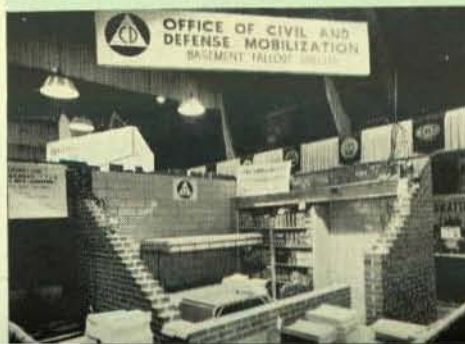
"Cut-away" view of home fall-out shelter was feature of exhibition shown by Office of Civil Defense.
