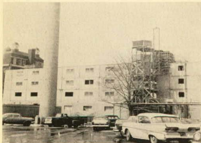
These members of Local 43, are wiring the new addition to the motherhouse of the Sisters of St. Francis in Syracuse, N.Y. This is one of the first multi-storied construction jobs of tilt-up precast walls. At right above are Foreman Carl Bauder and Brother Jerry Hart and below are Brothers Sam De Fonde, Willis Reese and Rovell Fuller.
