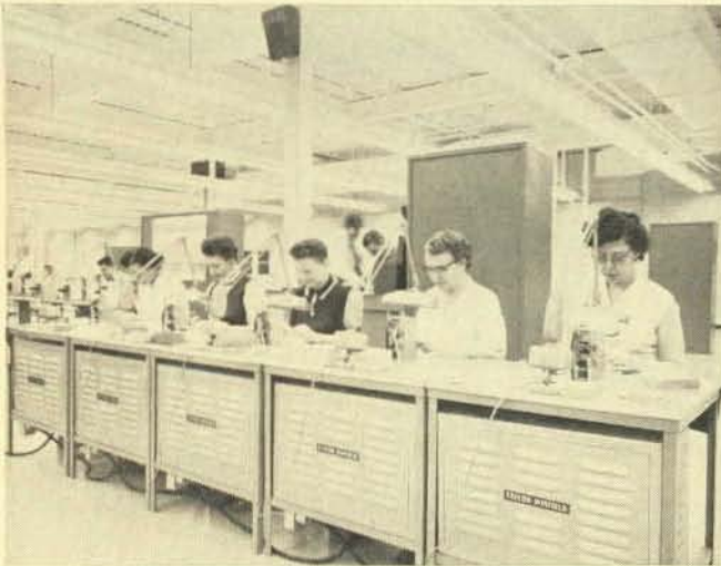
Hard at work at the RCA plant in Findlay, Ohio, are these welders, including (left to right) Helen Smith, Evelyn Balmer, president of Local 1907, Donedia Solomon, Thelma Smith and Helen Clark. At right, Local 1907 furnishes us with an operator's eye view of the welding operation on the transistors.
