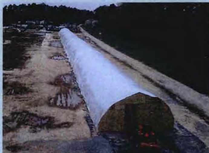
Figure 3. Engineered bioremediation cell (complete) at WPNSTA Yorktown
