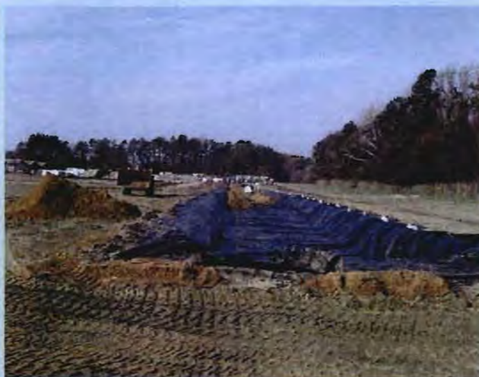
Figure 2. Engineered bioremediation cell (under construction) at WPNSTA Yorktown
