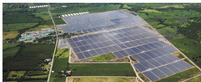
Fig. 3. LSP’s plant overview [7].
