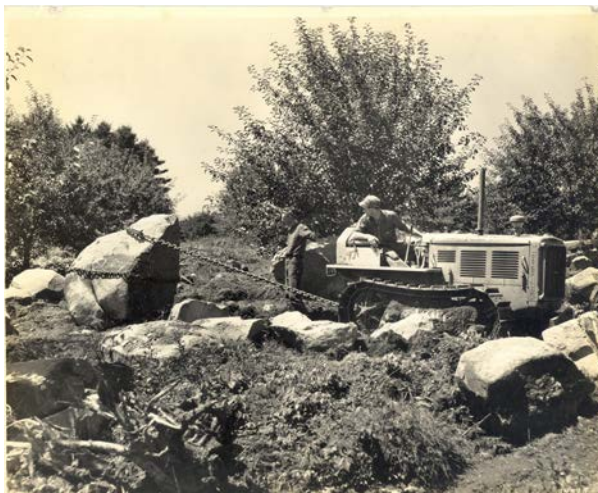
Figure 5-17. Photograph of bulldozer at work on the SBSB Site.
