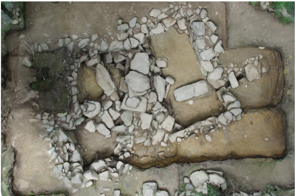
Figure 4-16. Overhead 3D rendering of the cellar foundation and drain, generated from multiple photographs.
