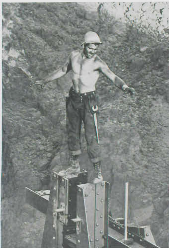
Steel Worker Atop Tower Far Above Boulder Dam
