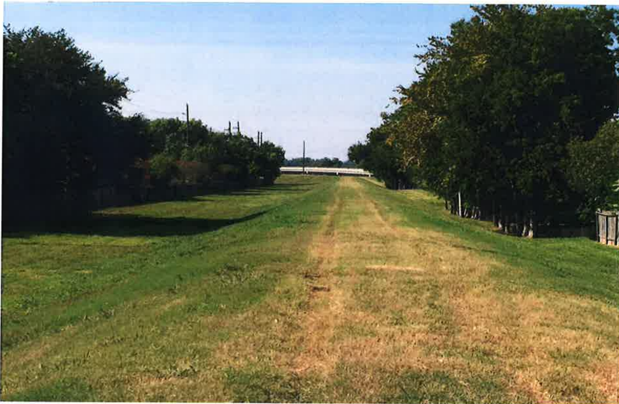
Levee South of Commonwealth Blvd.
