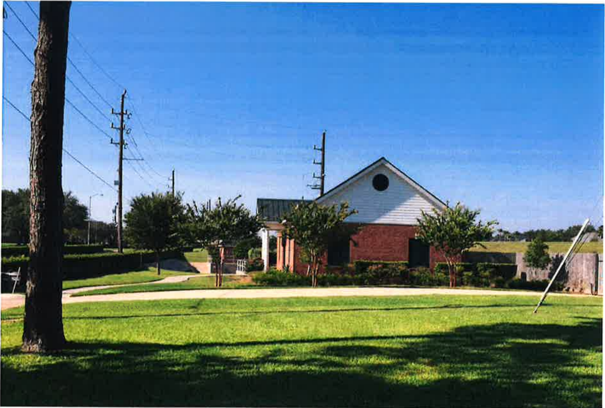
Pump Station Facility
