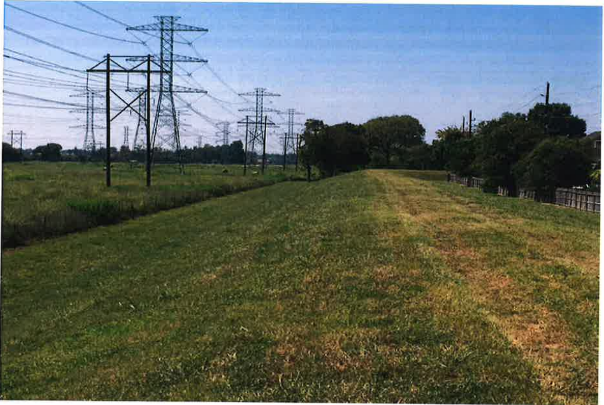
Southeast Section of Levee – South of Commonwealth Blvd.
