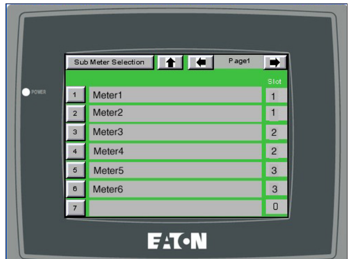
Figure 84. The System Sub Meter Screen.
