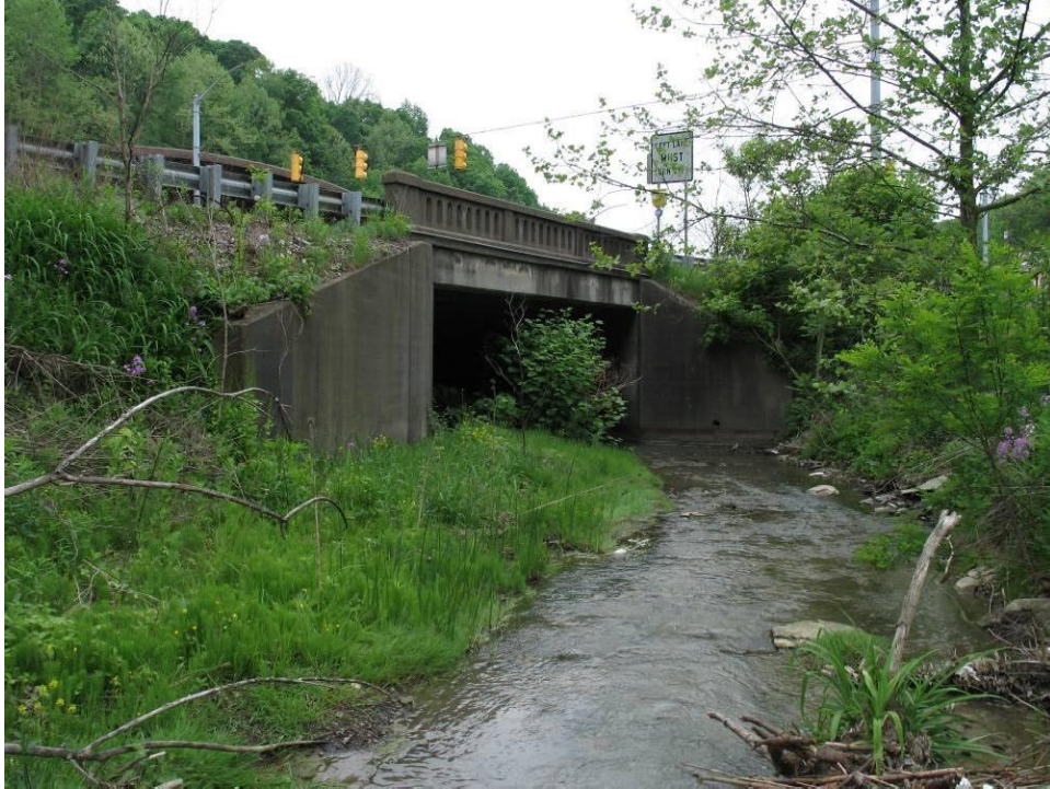
PHOTO NO. 13: Inlet of Bridge/Culvert Structure Upstream of Hutchinson Hill Bridge
