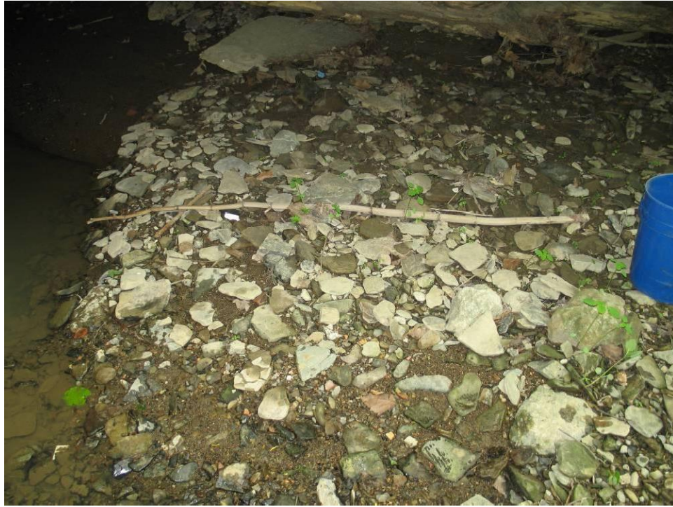
PHOTO NO. 25: Sediment Under Hutchinson Hill Bridge at Upstream End with Sand, Gravel, Flat Stones and Cobbles
