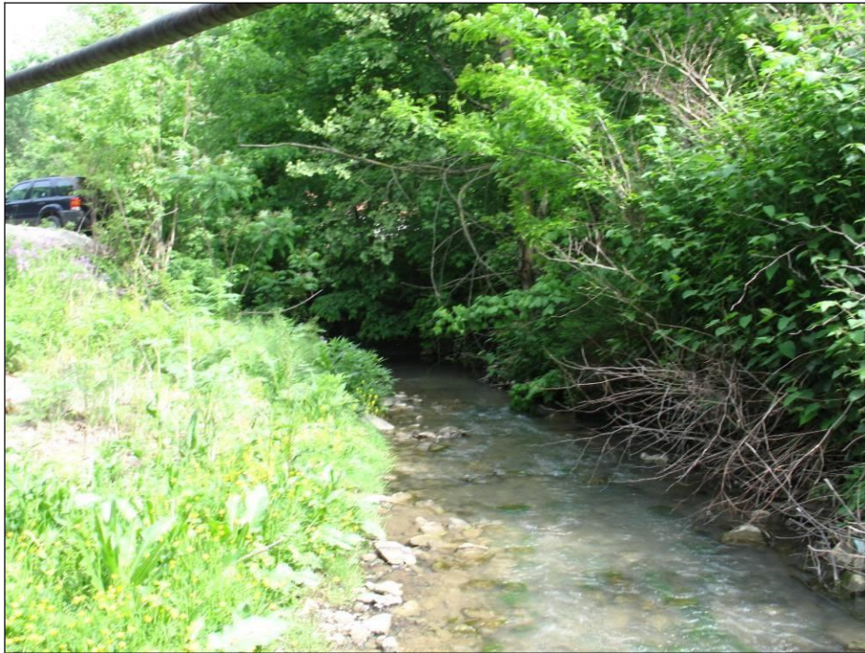
PHOTO NO. 6: Downstream Channel Seen from Hutchinson Hill Bridge Over Fallen Timber Run
