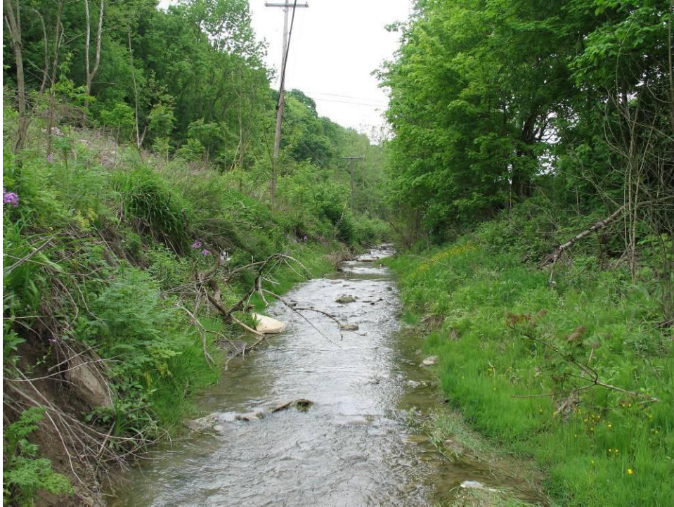
PHOTO NO. 15: Channel Upstream of Bridge/Culvert
