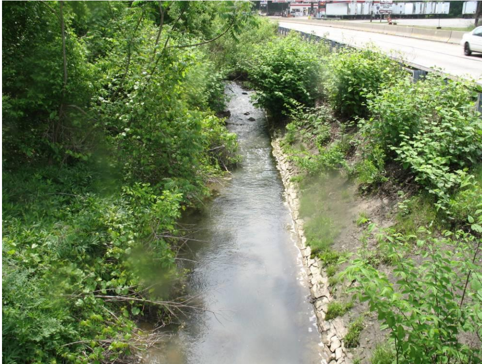
PHOTO NO. 22: Channel Upstream of Penneman Drive Bridge
