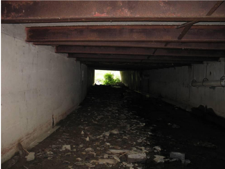
PHOTO NO. 14: Inside of Bridge/Culvert Structure Looking Upstream at Inlet
