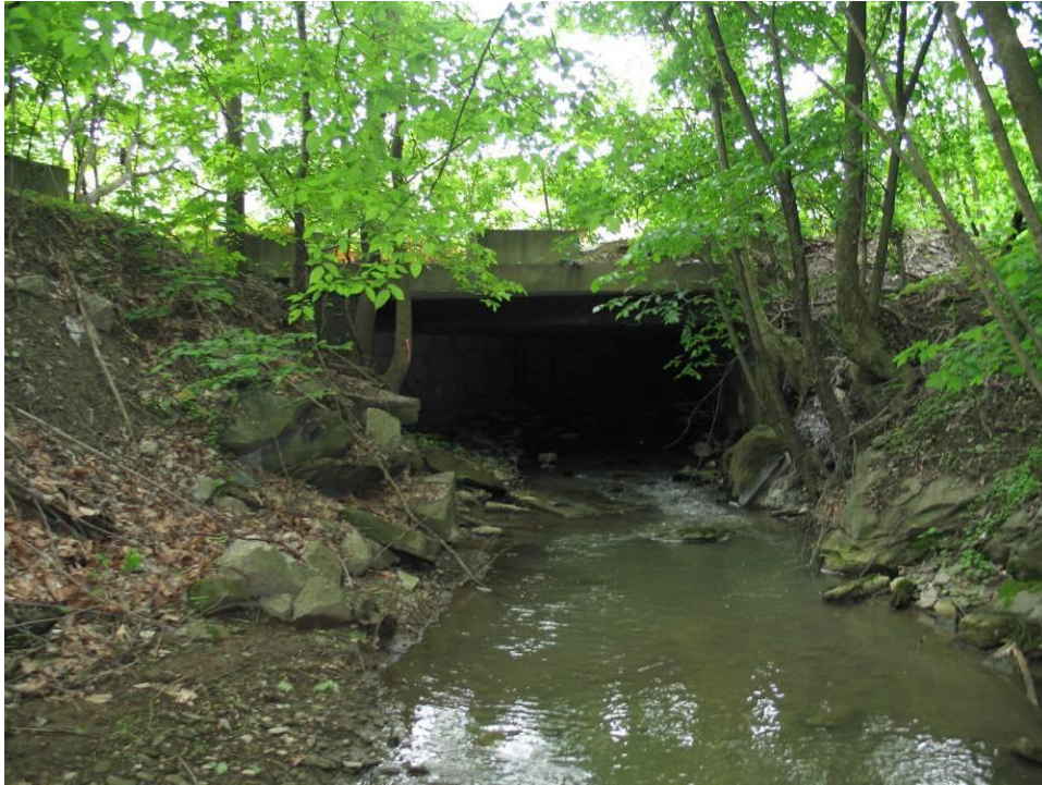
PHOTO NO. 12: Outlet of Bridge/Culvert Structure Upstream of Hutchinson Hill Bridge
