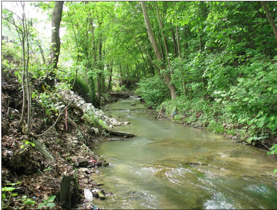
PHOTO NO. 4: Upstream Channel Seen from End of Right Wingwall of Hutchinson Hill Bridge Over Fallen Timber Run – Note Bedrock in Channel.
