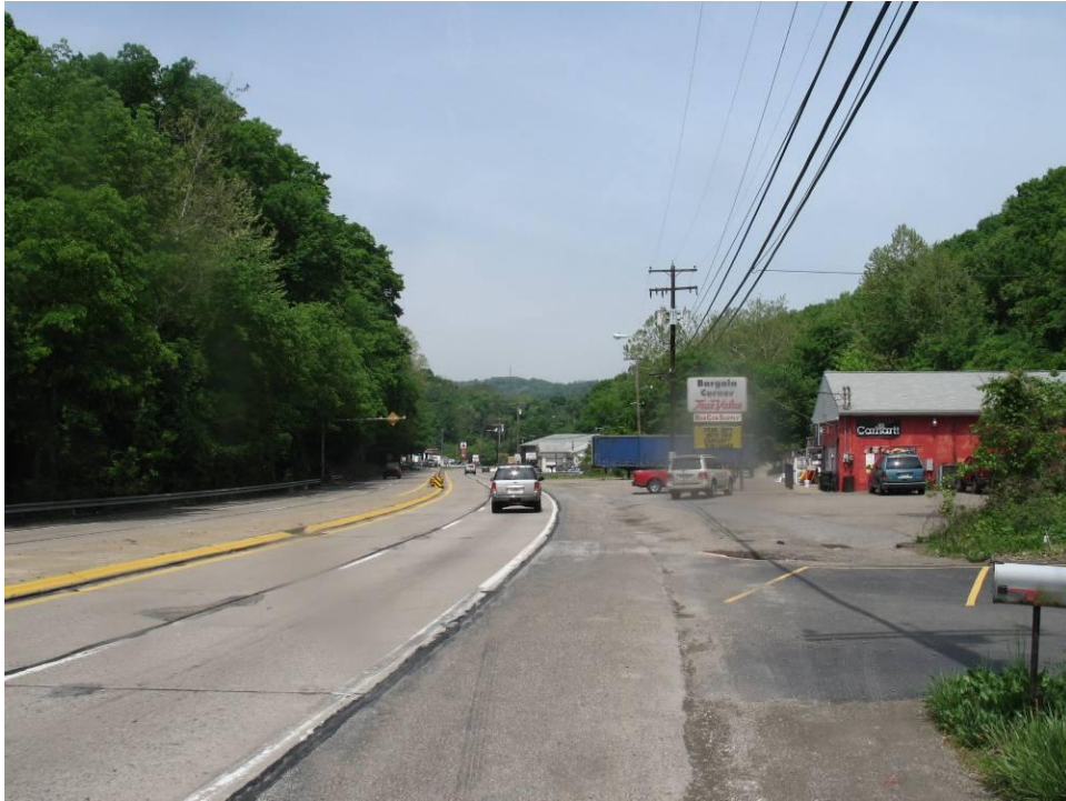
PHOTO NO. 16: Drainage Area Upstream of S.R. 051
