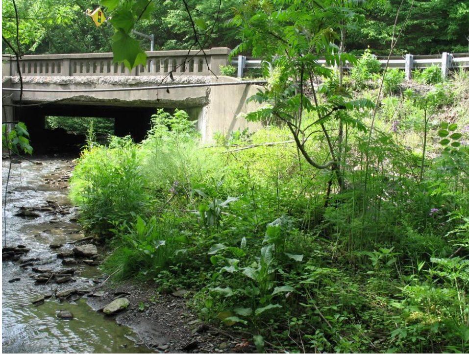
PHOTO NO. 17: Vegetated Sediment Accumulation at Left Side of Channel Just Downstream of Hutchinson Hill Bridge
