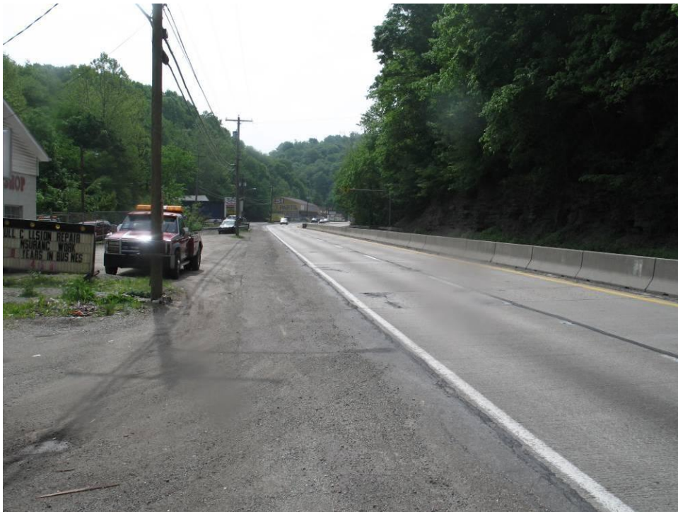
PHOTO NO. 2: North Approach Roadway (S.R. 51) to Hutchinson Hill Bridge (Facing South)
