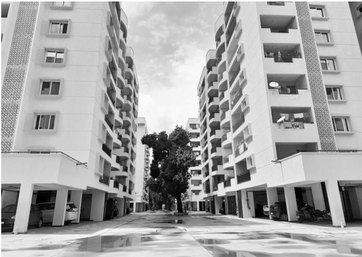
Multi - Storied Residential Quarters for M/s Bharat Electronics Ltd at Bengaluru
