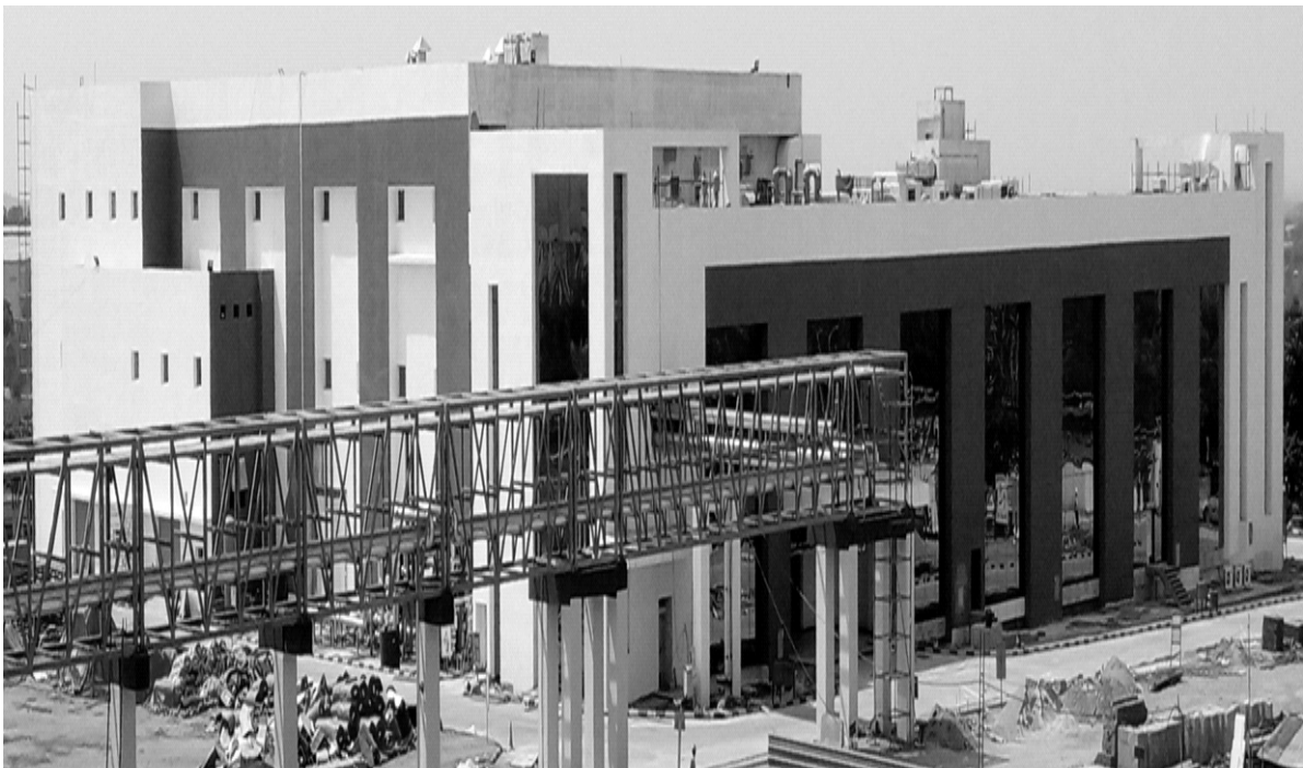
New Insuman Cartridge Enterprise [NICE] building for M/s Shantha Biotechnics Private Limited (A Sanofi Company) at Muppireddypally, Hyderabad
