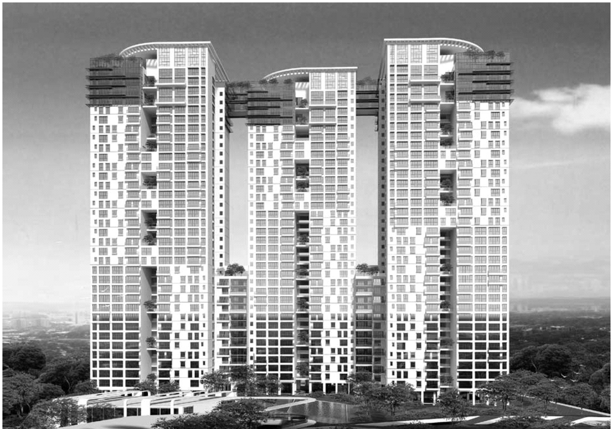
Karle Zenith Towers at Bangalore (3 Towers each of 3B+G+35Floors)
