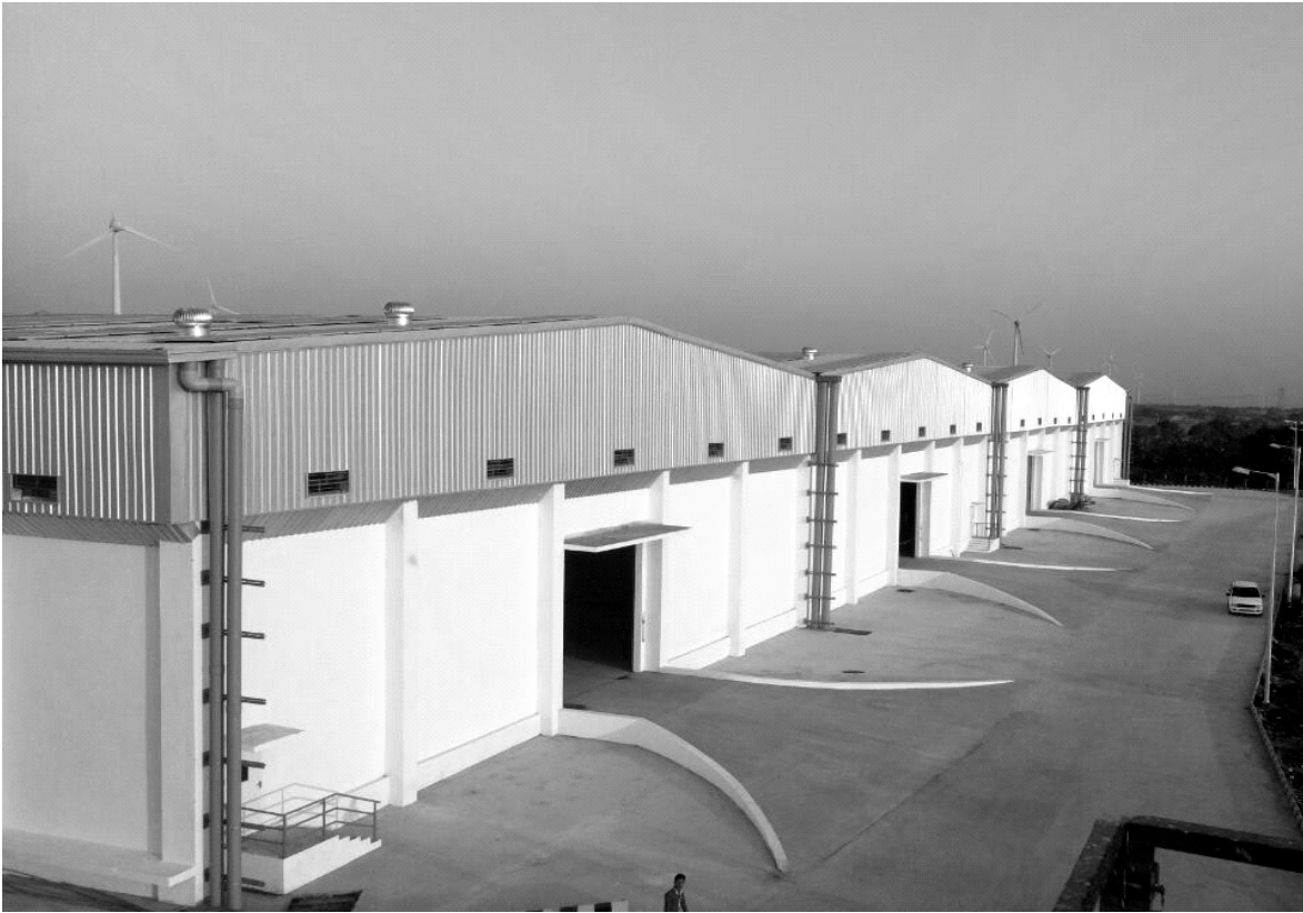
Warehouses for M/s Hatsun Agro at Palani, T.N (Project Completed in 110days)
