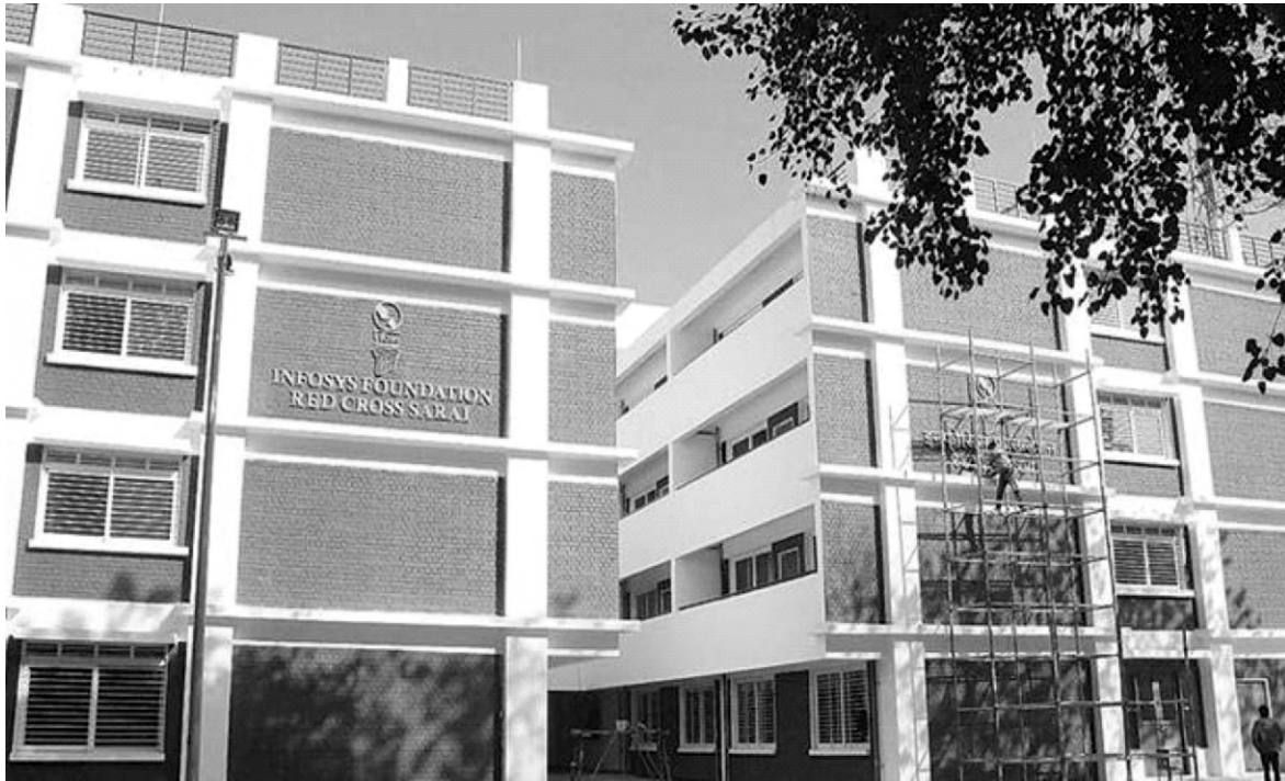
Red Cross Sarai - Dormitory Building at Chandigarh for M/s Infosys Foundation
