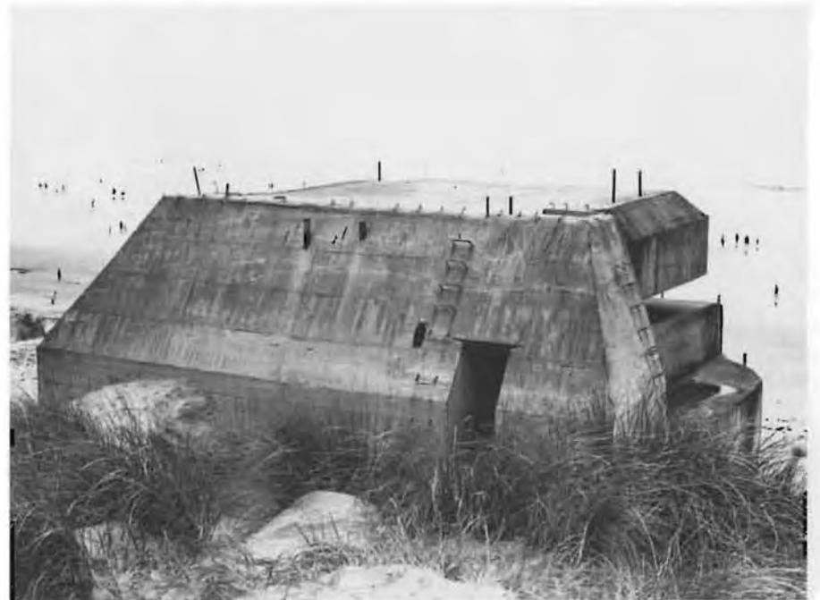
EXPERIMENTAL MOBILE BUNKER: THE UPPER MASS PIVOTS ON ITS BASE
