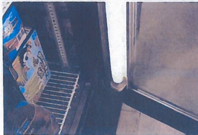
Case lighting is fluorescent.
