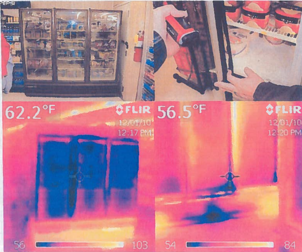
The case on the right has good seals and glass. The case on the left has a damaged seal that allows cold air to leak out on the floor.
