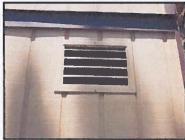
Examples of fresh air intakes at your church
