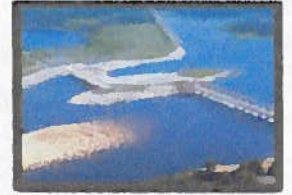
Electric Cooperatives of Arkansas Hydropower Generating Station
