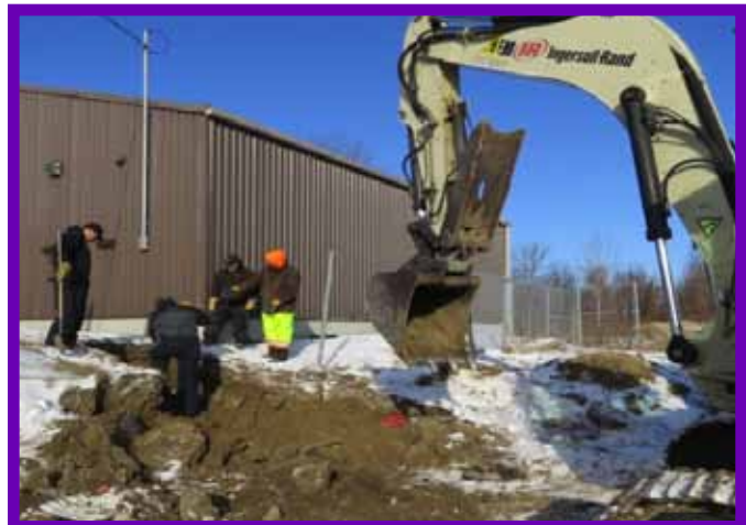
Waste and Wastewater rerouted the piping inside the plant
