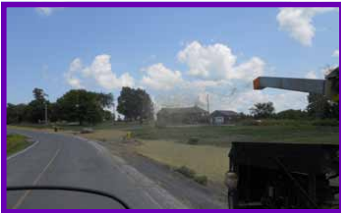
Contract 3-Tsi Snaihne Water Supply Project
