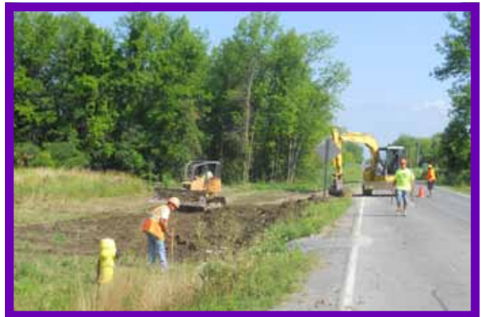
Contract 2-Tsi Snaihne Water Supply Project
