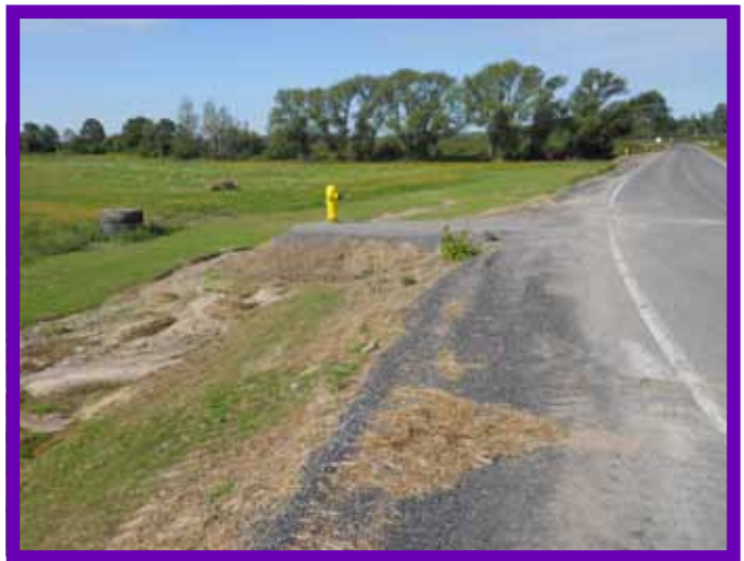
Contract 2-Tsi Snaihne Water Supply Project
