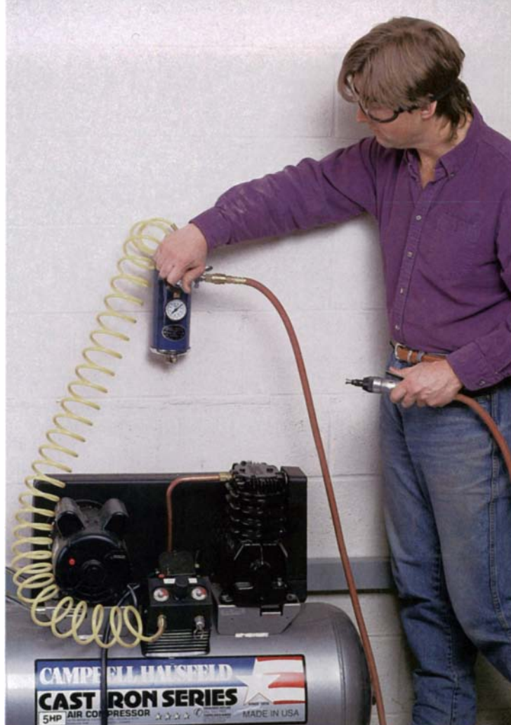
A large air compressor can drive many pneumatic tools, including air sanders and die grinders. The author adjusts the pressure regulator on a wall-mounted air-filter unit, which is connected to the compressor by a flexible plastic hose.
