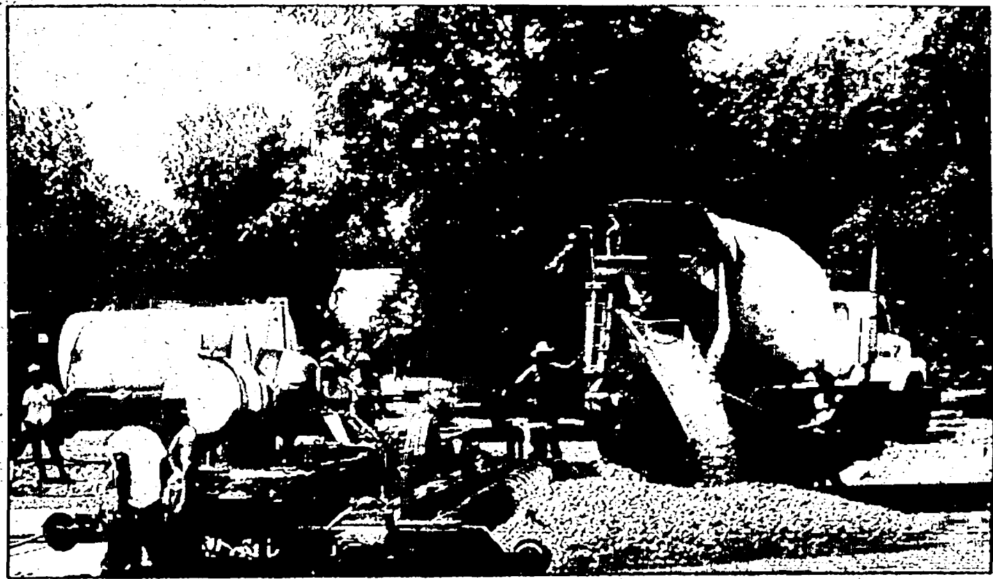
Road crews worked in 90-degree weather last week to pour the new Newburgh concrete.
