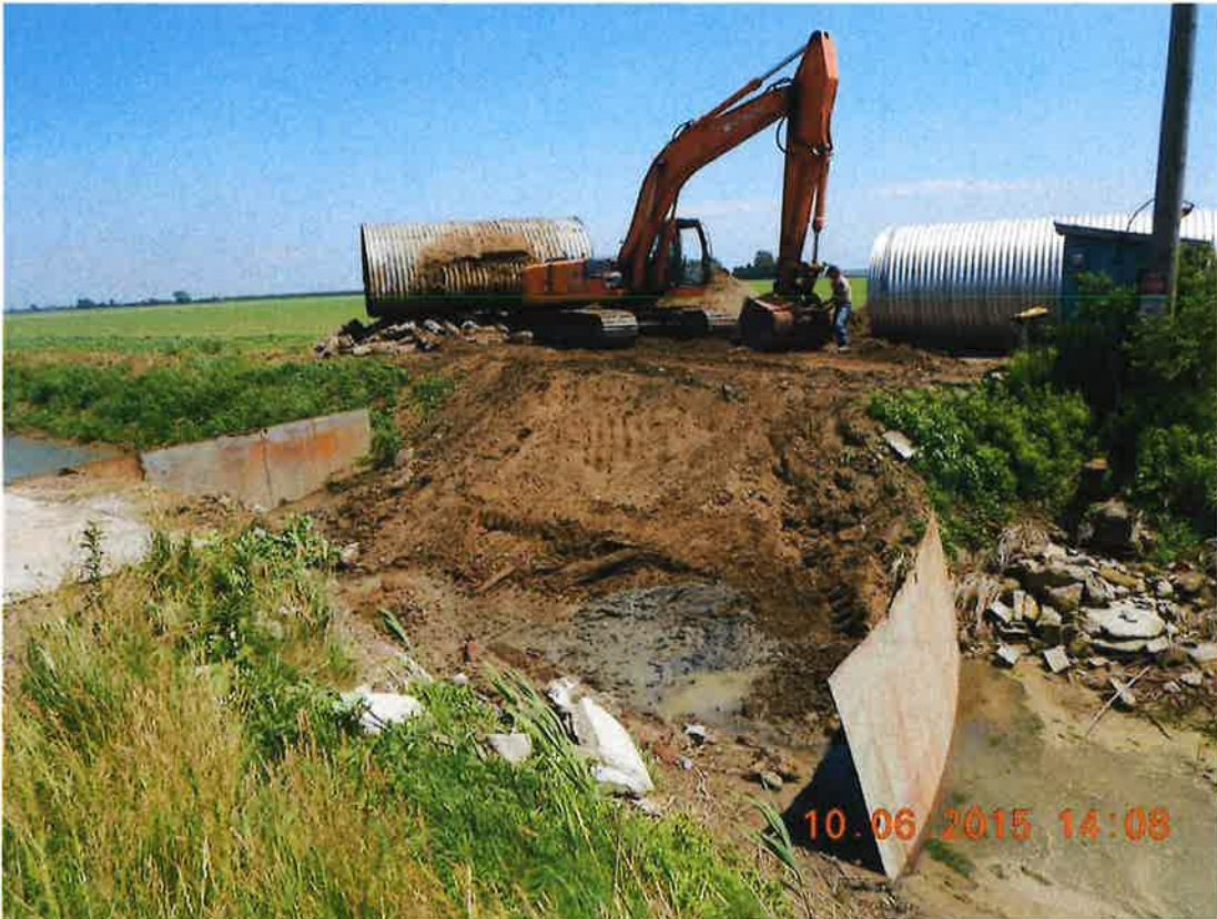
Figure 2. Isolation of Site
