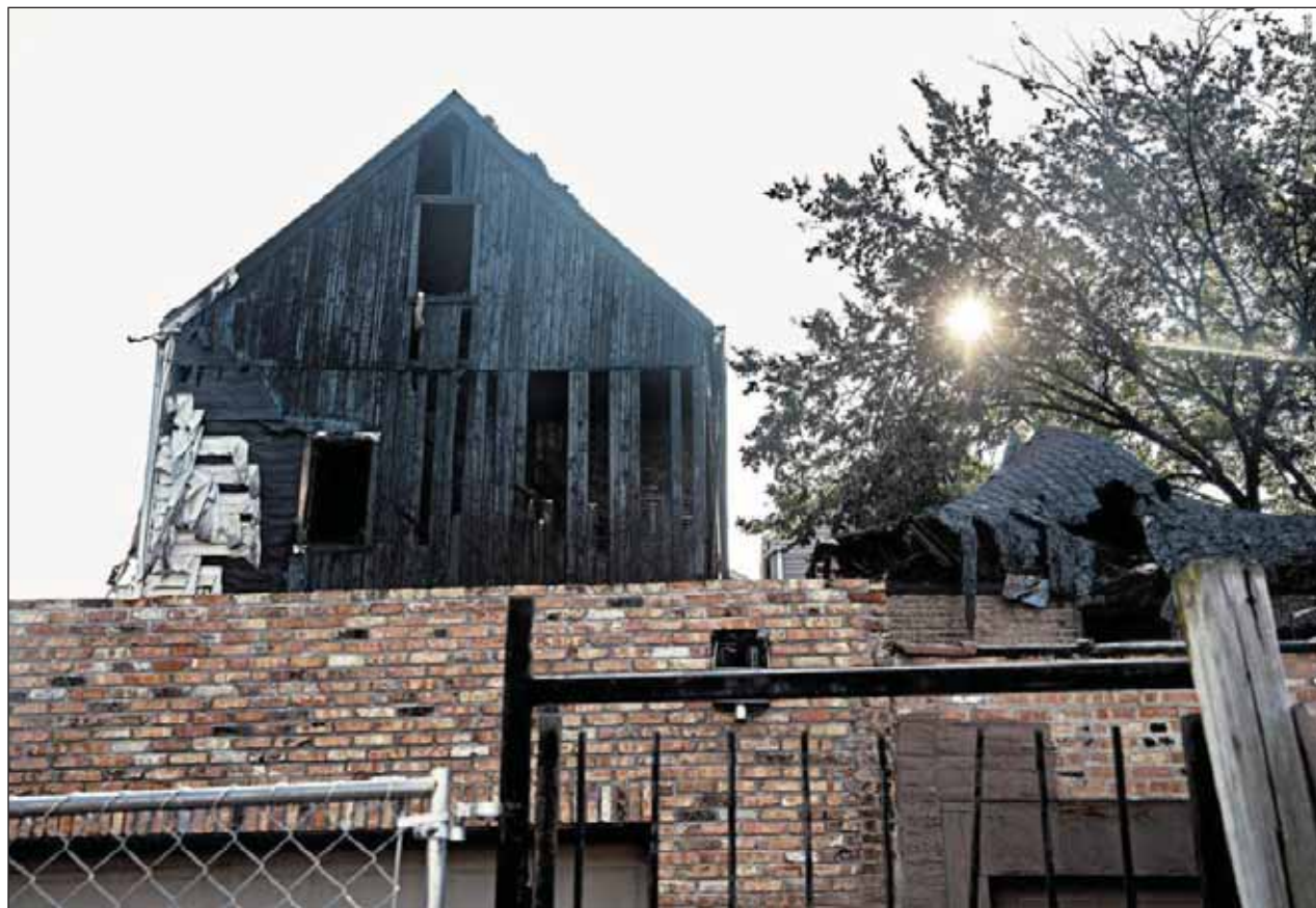
The fatal fire in the 2200 block of South Sacramento Avenue spread to several nearby homes and buildings.
