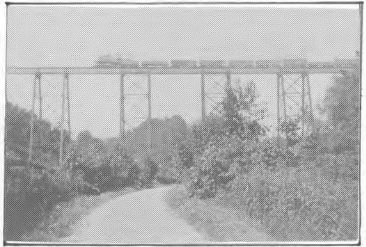
New York Central Freight trains crossed Tinkers Creek Valley on this trestle-supported bridge. The freight line operated from 1911- into the 1960s
