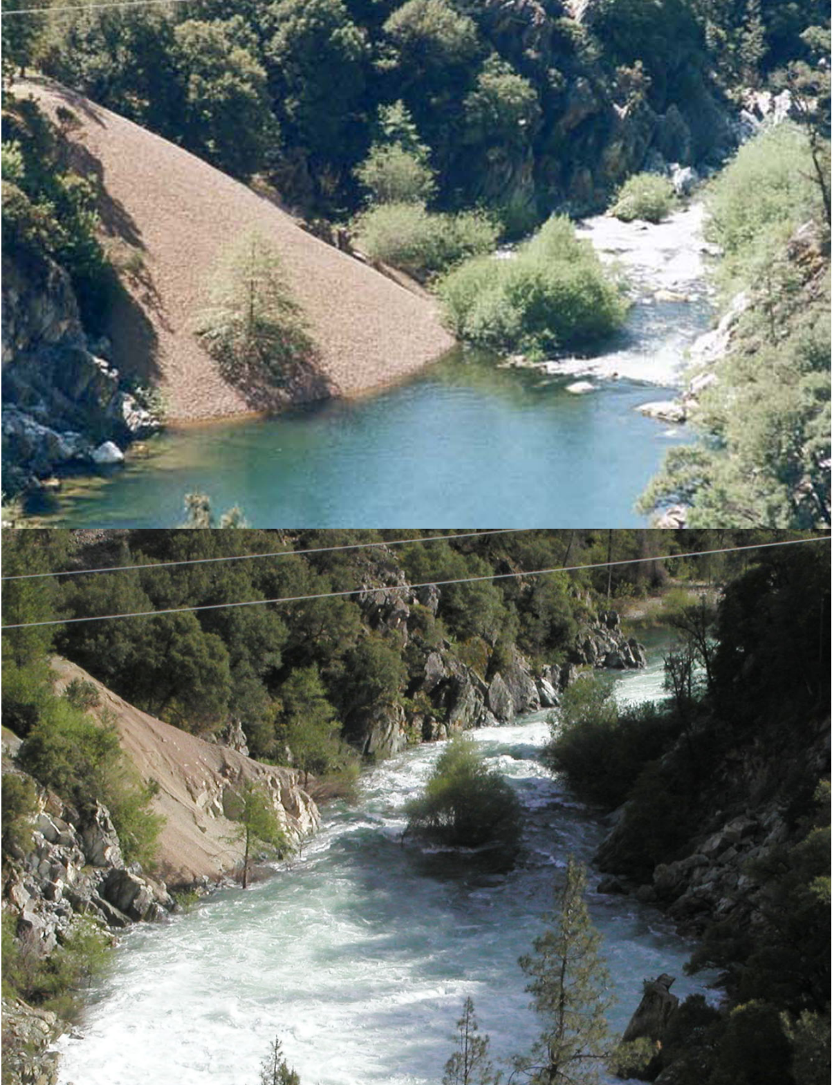
Figure 26. Coarse sediment introduction below Whiskeytown Dam on Clear Creek, near Redding CA, using the high-flow recruitment method, with gravel end-dumped from the hillside above. The top photo is from April 2000. The bottom photo, from May 2003, shows most coarse sediment having been mobilized during intervening high flow releases from Whiskeytown Dam.
