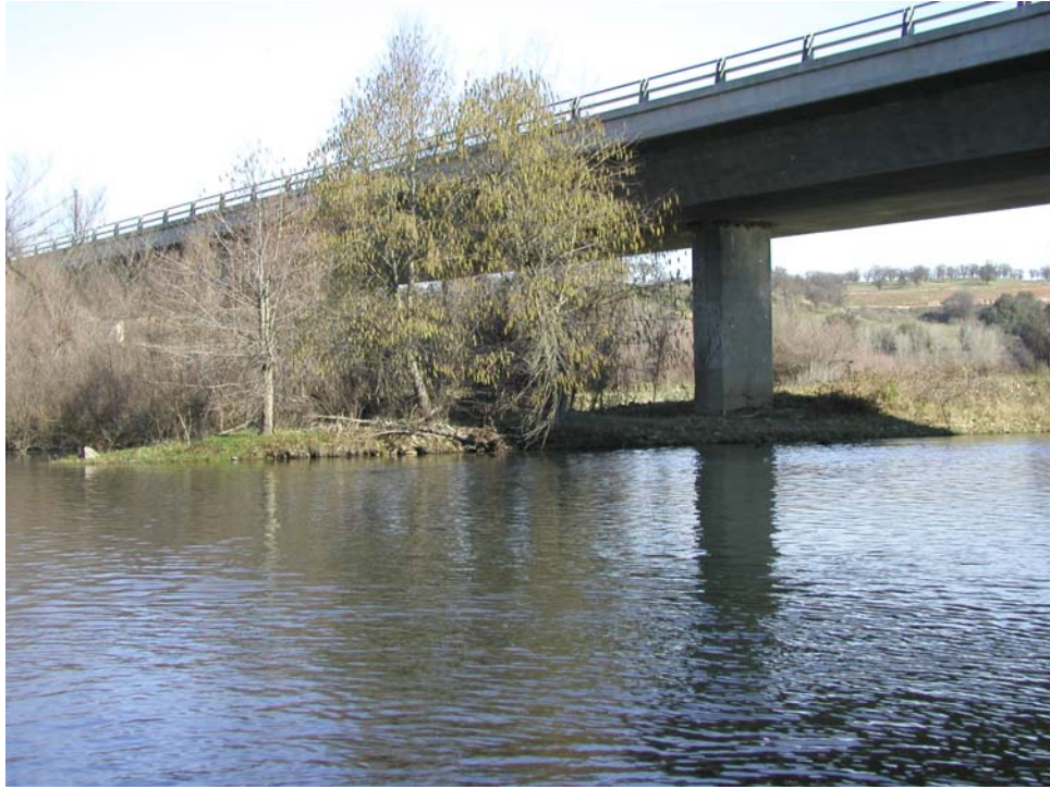
Photo 5. Site #7 (J59 Bridge)
