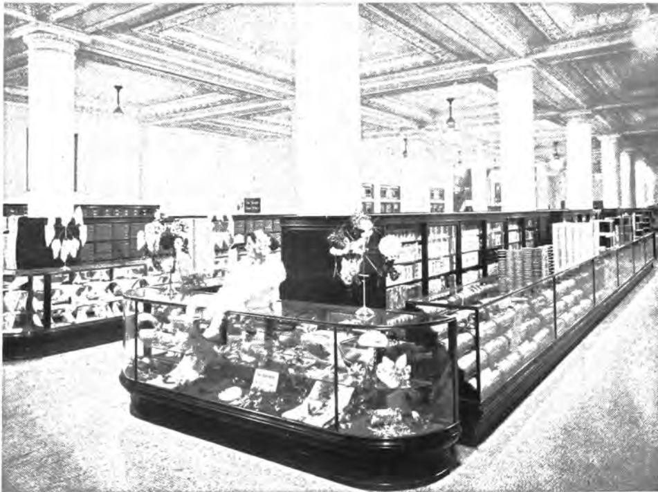
Store Lighting with Intensified Arc Lamps, R. H. Stearns' Store, Boston, Mass.
