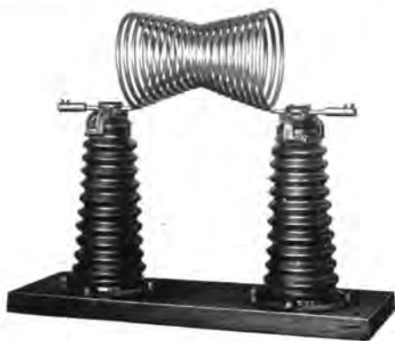
HOUR GLASS TYPE—CHOKE COIL 15000-35000 VOLTS
