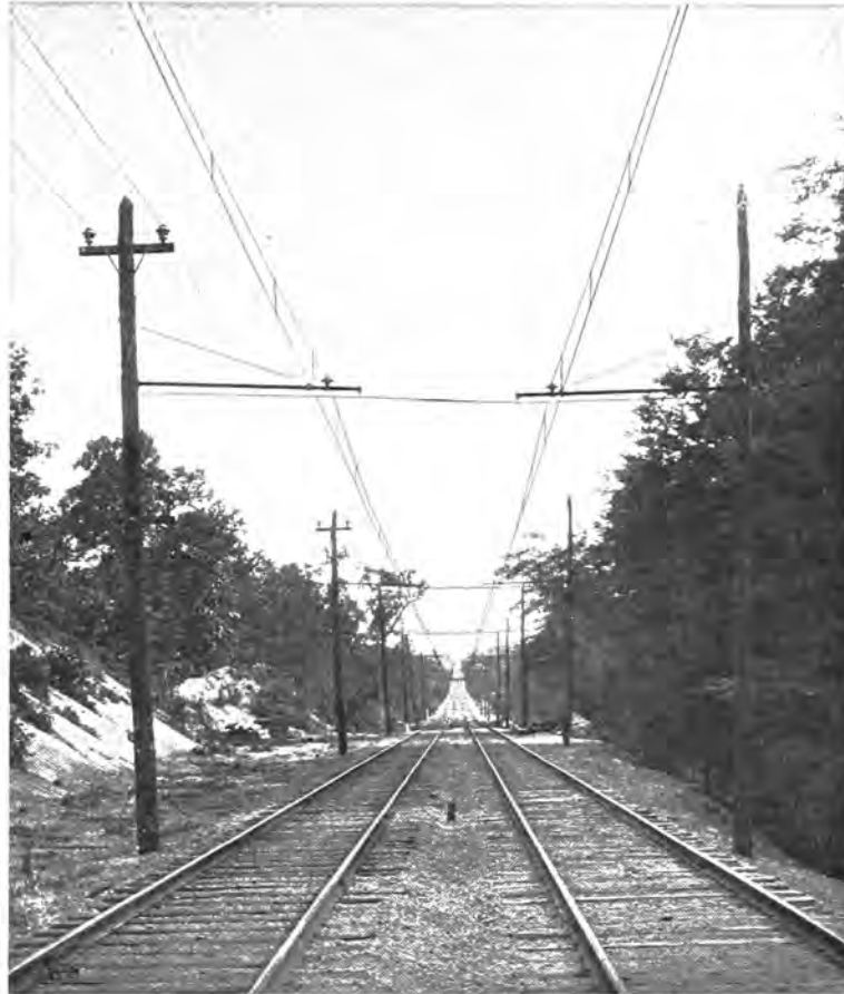
Catenary Line Construction on the Washington, Baltimore and Annapolis Railway
