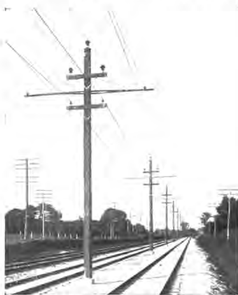
Double Track Tangent Construction
