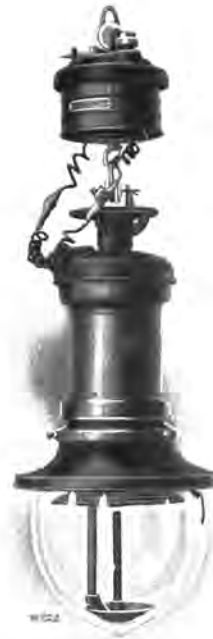
Power Circuit Multiple Luminous Arc Lamp with External Cutout Resistance
