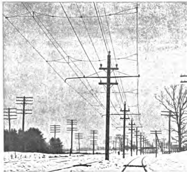
Double Track Pull-Off with Bracket Extensions
