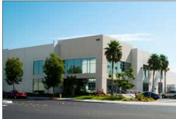
World Headquarters, Los Angeles, USA
