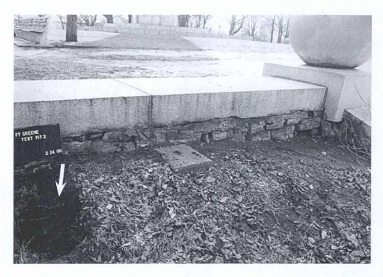
16 Test Pit 2 (TP2, arrow), a shallow test near the plaza steps (right). This test was terminated when tubing and roots were encountered close to the surface. Note the exposed brick under the wall's coping, a focus of the reconstruction. (Geismar 2/24/00)
