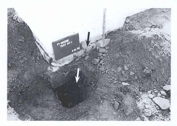
15 Test Pit 1 (TP1, white arrow) outside the north corner of the memorial plaza. The excavation extended down 3.2 ft. below granite base. Note exposed brick (black arrow) under the base. (Geismar 2/24/00)
