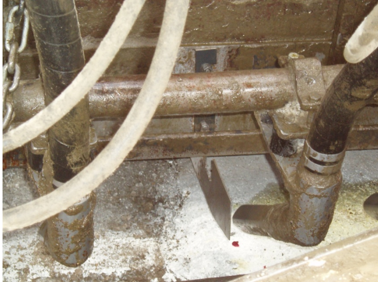
Figure 35. “Knife” mounted on the bottom of the slipform paver pan
