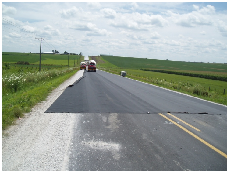
Figure 26. Fabric and concrete placement
