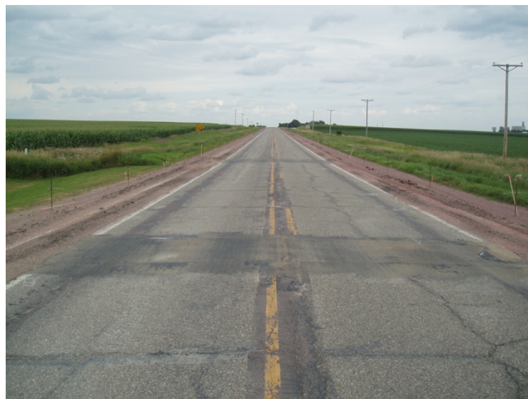
Figure 9. Osceola County original pavement
