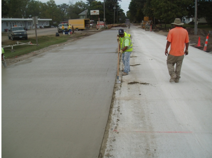
Figure 16. Hand tooling of the center line
