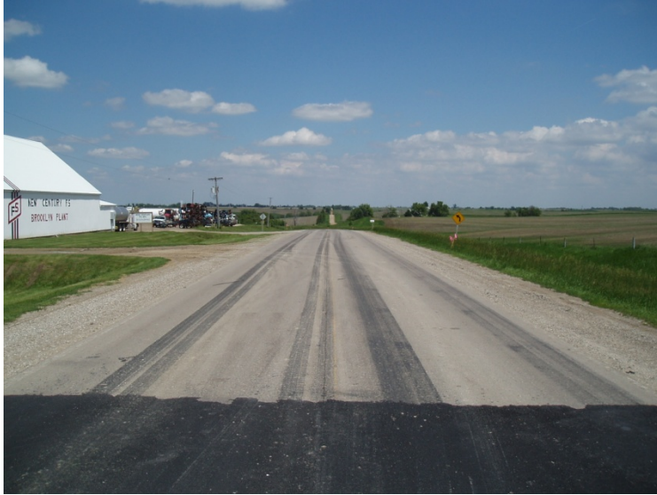
Figure 27. Poweshiek existing pavement
