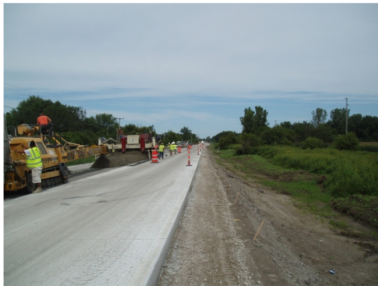
Figure 29. The project paving train
