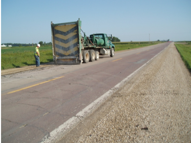
Figure 13. Worth County before milling
