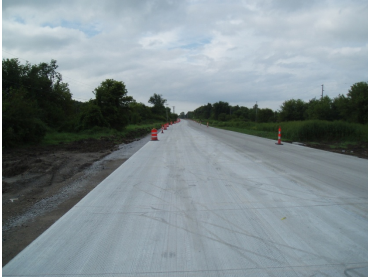
Figure 30. Johnson County finished pavement
