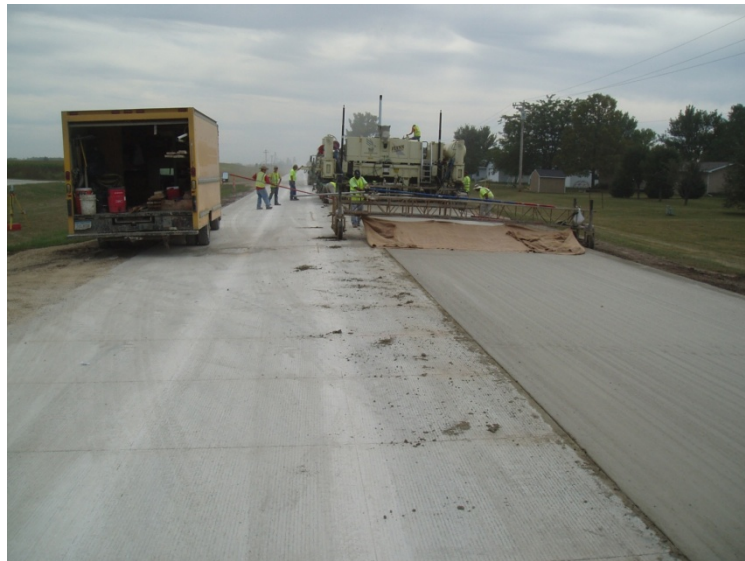
Figure 10. Mainline paving
