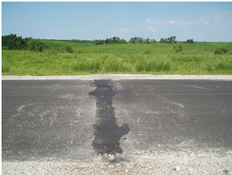
Figure 28. Rehabilitation technique for damaged transverse joints
