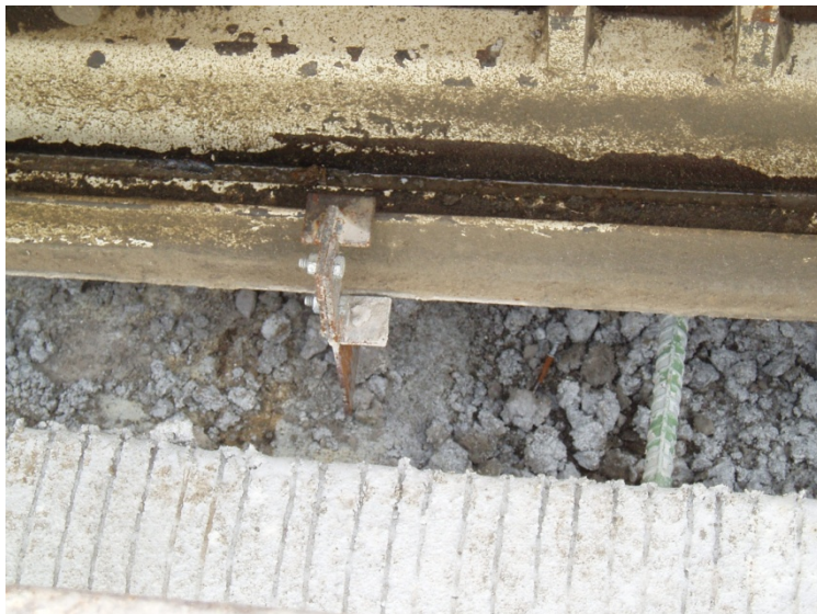
Figure 36. “Knife” held in place with clamps
