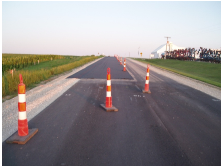
Figure 25. Non fabric-covered lane
