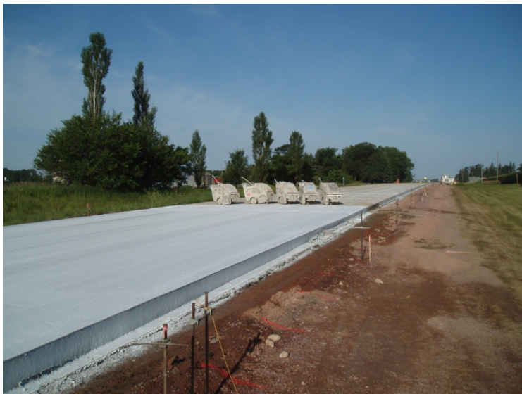
Figure 8. Osceola County finished pavement
