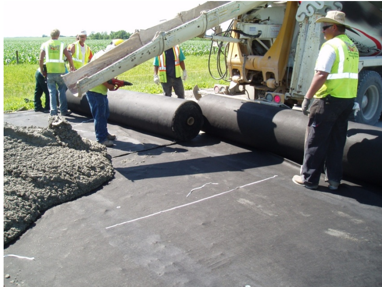
Figure 23. Unrolling and nailing the material to the existing pavement
