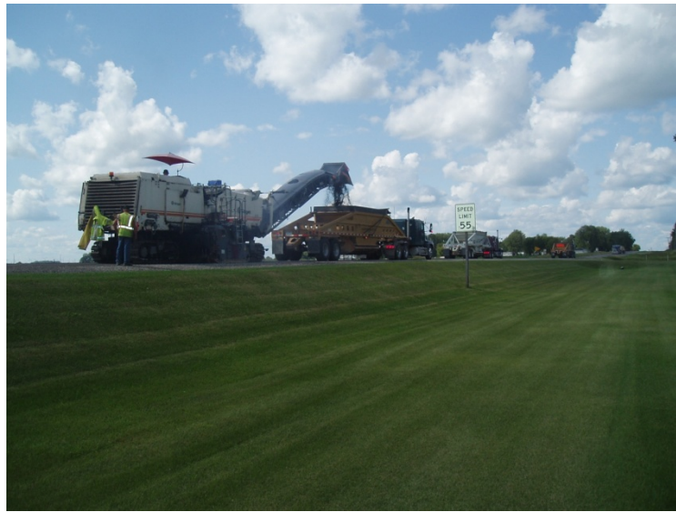
Figure 15. A 12-foot-wide milling machine
