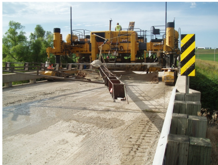
Figure 17. Gomaco 2800 Commander slipform paver
