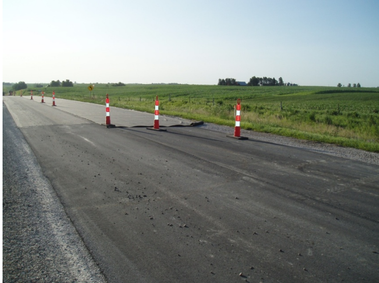
Figure 21. Fabric roll placement
