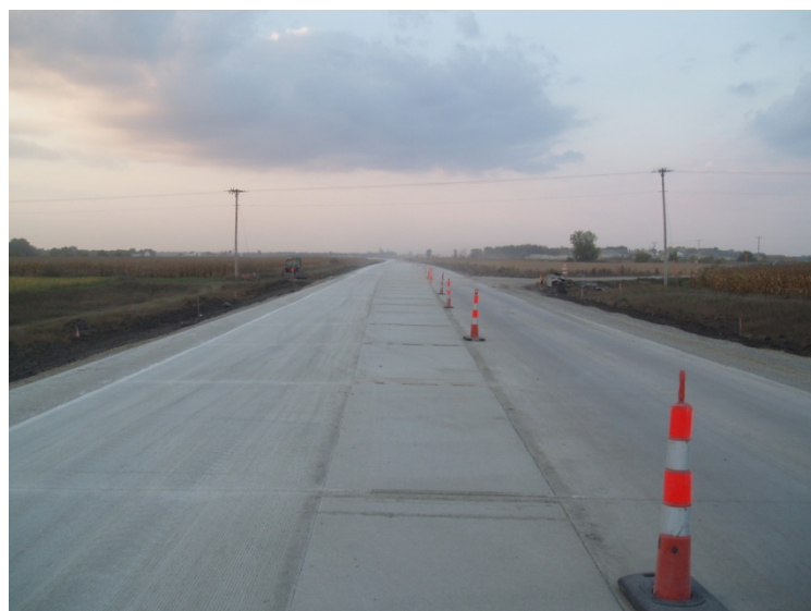
Figure 11. Worth County finished pavement
