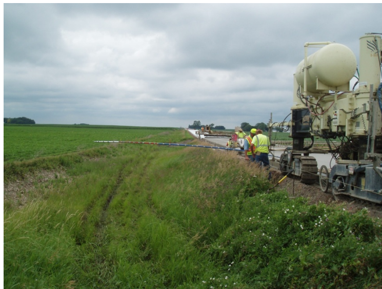
Figure 6. Osceola County paving train
