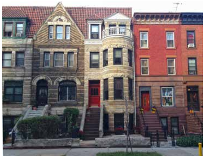
1199 Bergen Street (middle with rounded bay), Crown Heights North Historic District, Brooklyn
